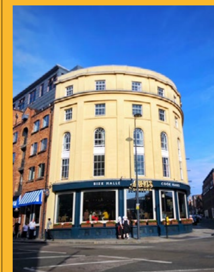
Casartelli Building before and after restoration
