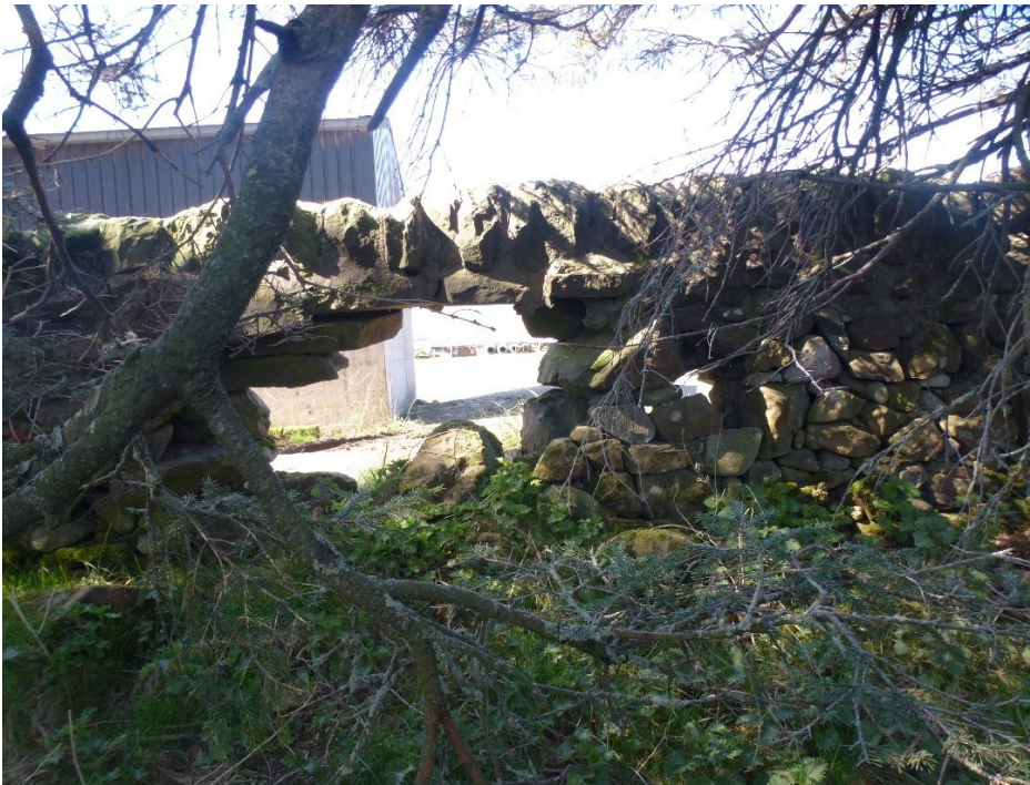
Photo 9: One area of damaged wall to west boundary.
