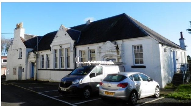
From West showing Church Road elevation
