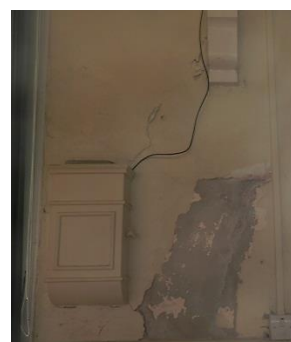
Dampness to wall
