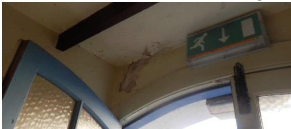
Damp above front entrance door
