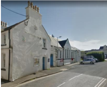
North East elevation from Main Street
