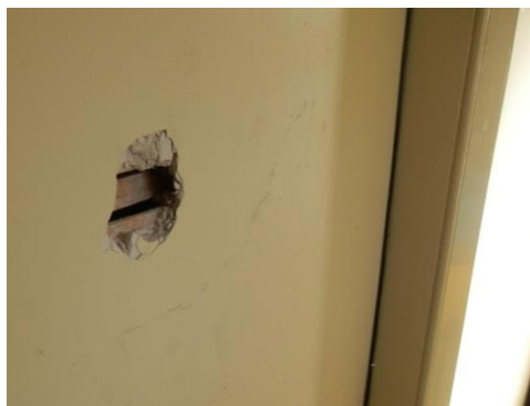
Green rooms – deteriorated paintwork and damaged plaster
