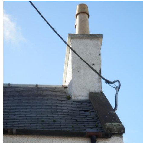
Right hand chimney stack to NW elevation
