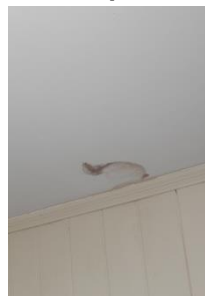
Damp at SE end
