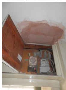
Repair – historic damp?
