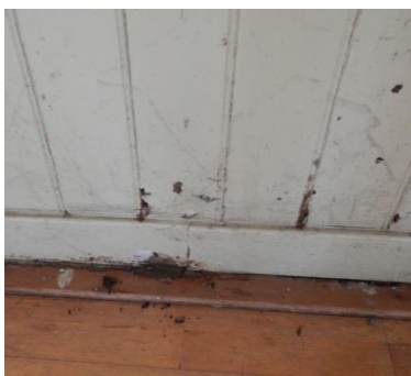
SE wall dampness under skirting
