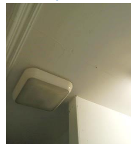
Crack above stairwell
