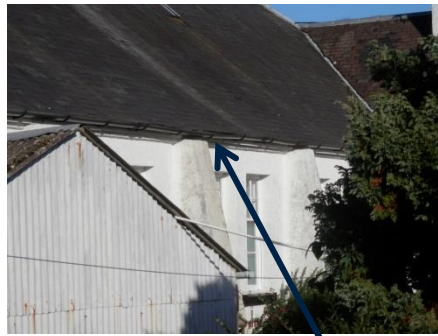
Central section of elevation with dipping gutter
