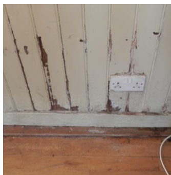
Dampness in timber boarding
