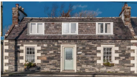
C-Listed property showing regular pattern of 3-bay frontages
