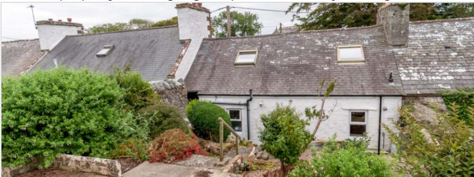
Rear view of part of terrace of C-Listed properties in Main Street, Mochrum
