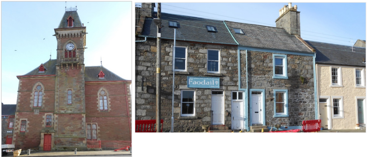
Wigtownshire County Building B-Listed C19 th
