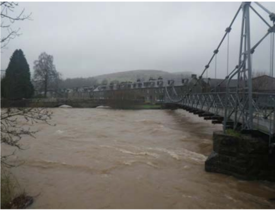
I – Looking upstream on Wauchope Water from George Street
