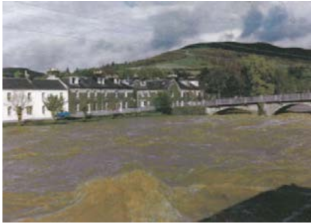
B: Looking upstream from George street
