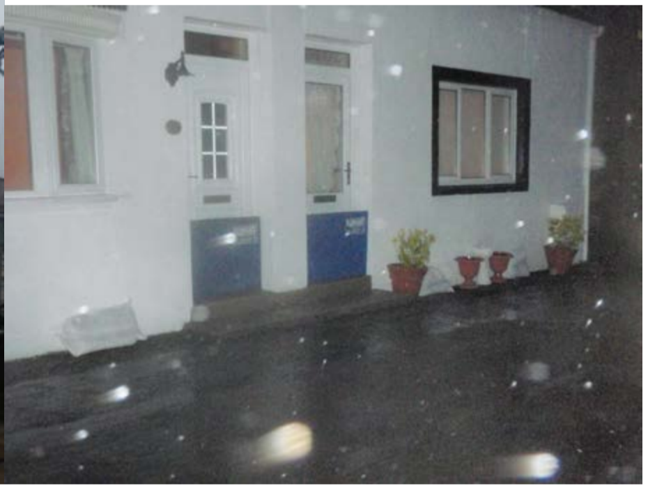
J – Flood gates installed on residential properties on George Street
