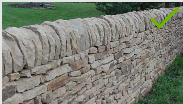
Dry stone wall with or without additional wire fencing
