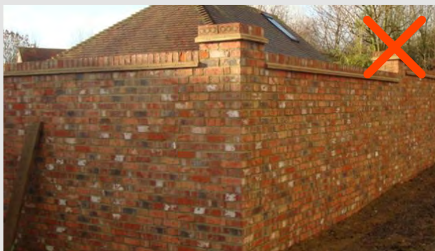
Brick 1.8m high boundary wall
