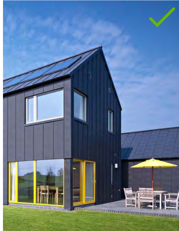
Aim for contemporary semi-rural character – Fordhouse in Castle Douglas by Simon Winstanley Architects
