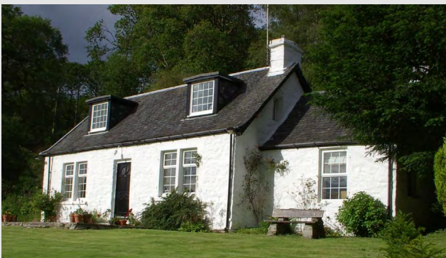
Typical 2 bay 1.5 storey cottage with extension – Gartmore
