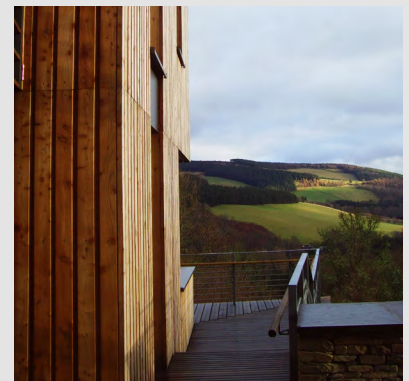
Timber cladding (Gaia Architects)
