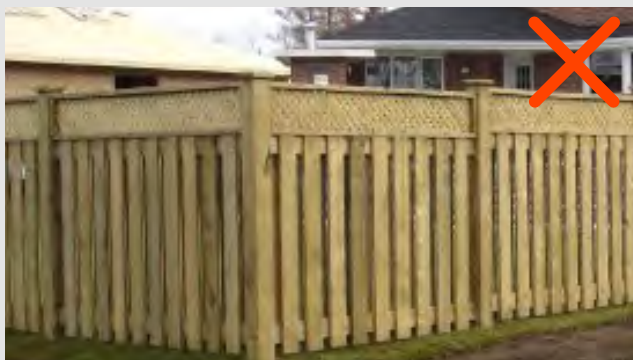
High timber fencing with solid appearance
