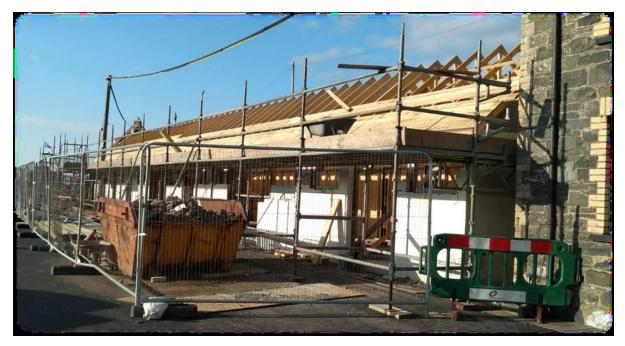
Below you can see work in progress with the new slate roof under construction
