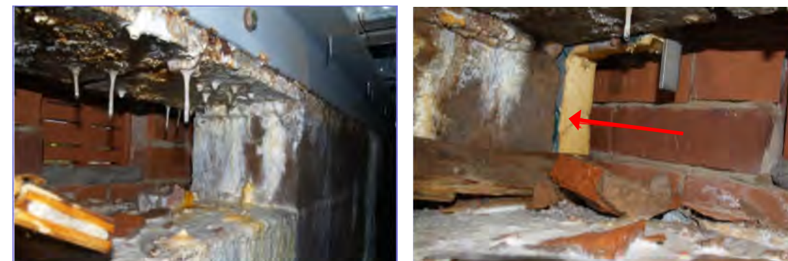
Saturated damp and efflorescence in void under pool area
