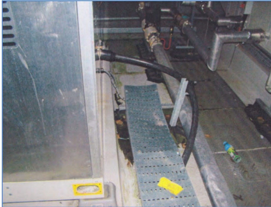
"Electric containment trays are being damaged by foot traffic and should be protected". H&K 2011
