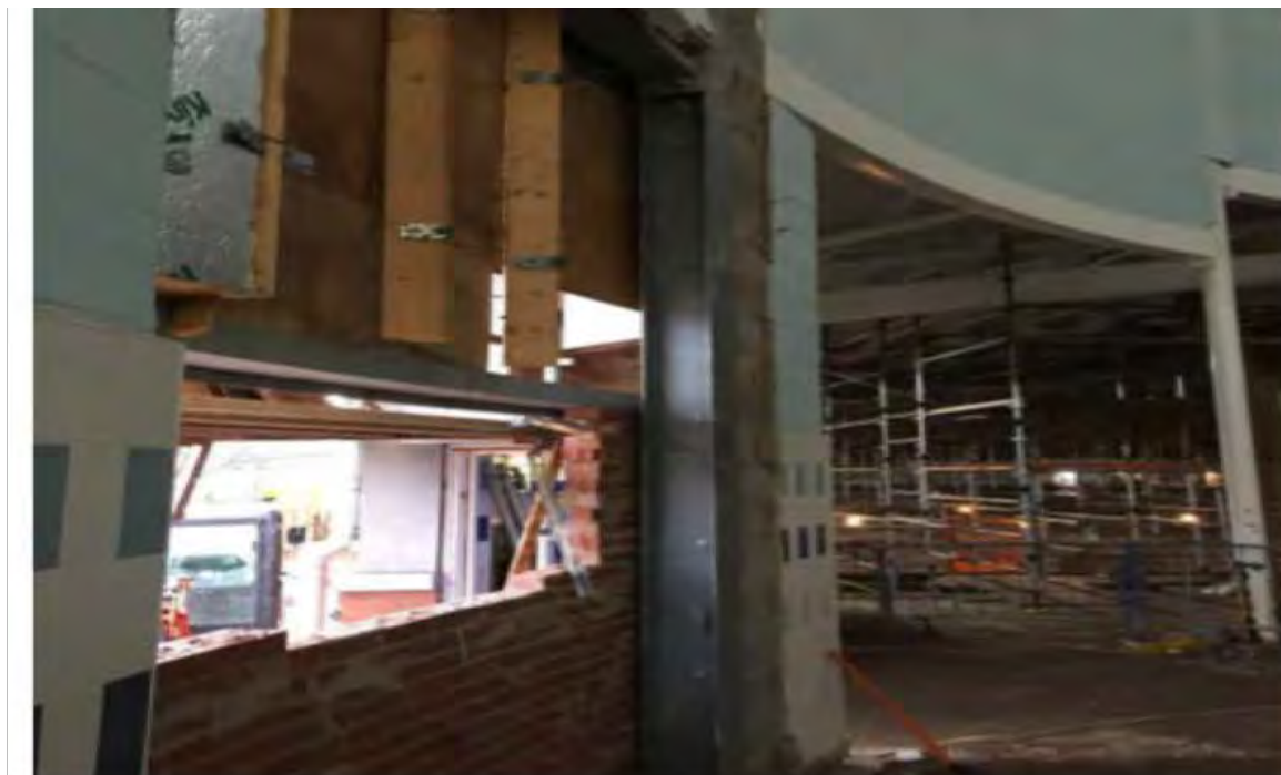
Piers 6. Wall panel in course of break out - inadequate wall tied to column and between external and internal leaf. External timber studs show fixings to single block leaf..
