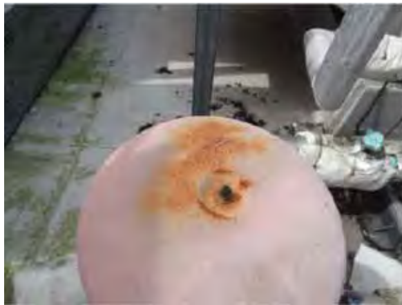
Corroding expansion chamber and valve
