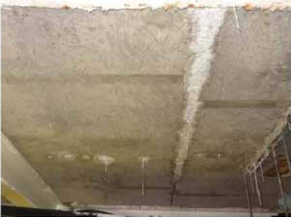
Leaks and lack of fire stopping
