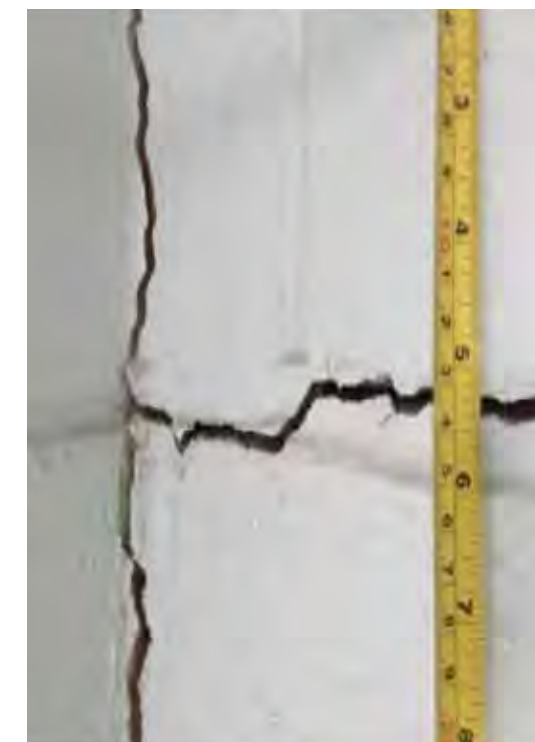
Piers 2. Block encasement removed. No ties in bottom 10 joint to left sides. No ties at all in right hand return. No ties to RHS of column in top section
