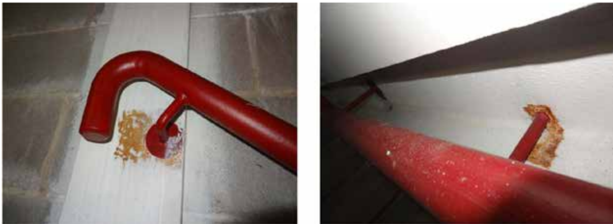
Corrosion to handrail support in escape stair.
