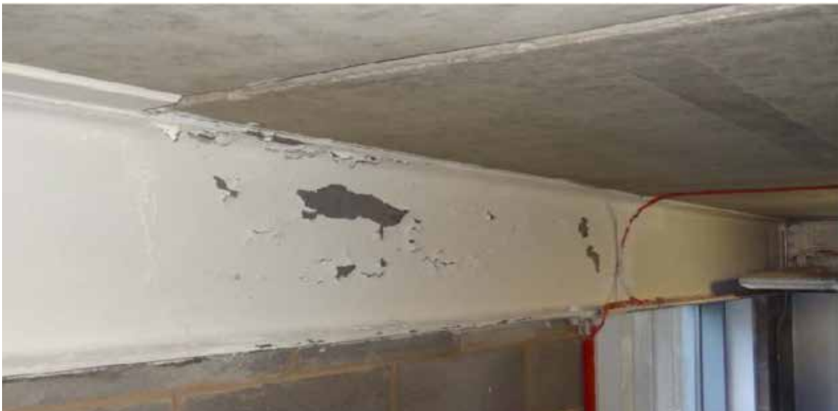
Failure of paint system
