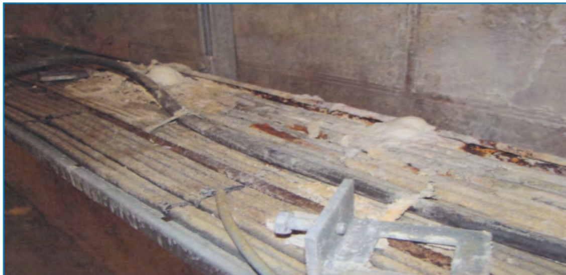
“Severe corrosion evident to electrical and mechanical services from pool chemicals and condensation”. H&K 2011
