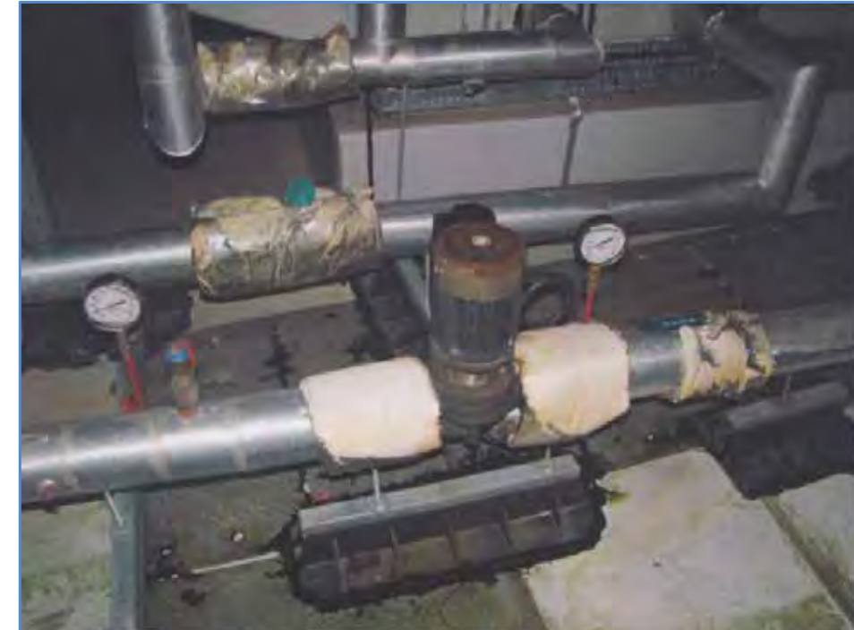
"Damaged insulation and corrosion to pump on roof" H&K 2011 allowing water to pond". H&K
