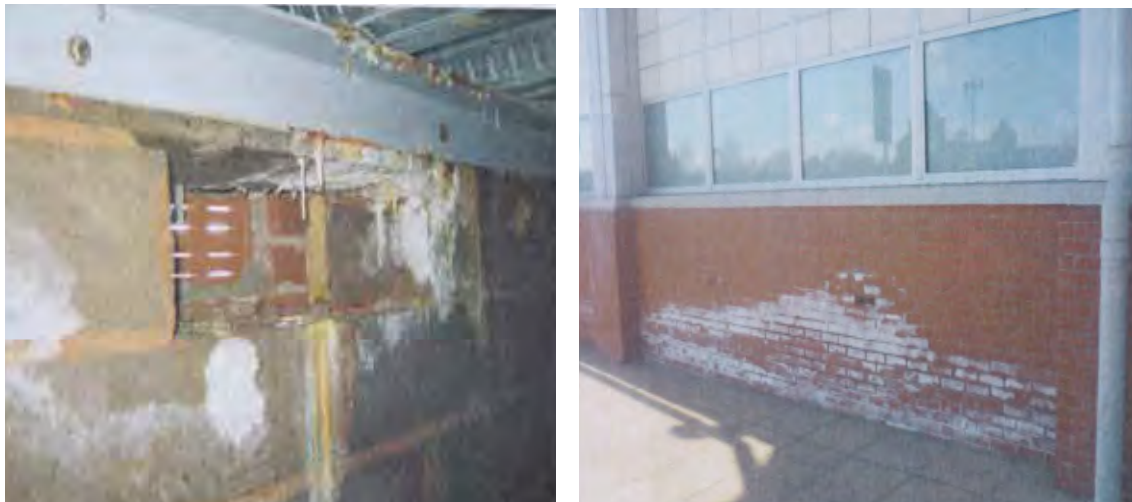
External and internal faces of saturated cavity wall
