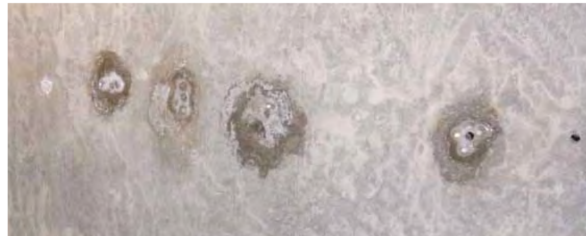
Water dripping from holes drilled in soffit of bison slabs
