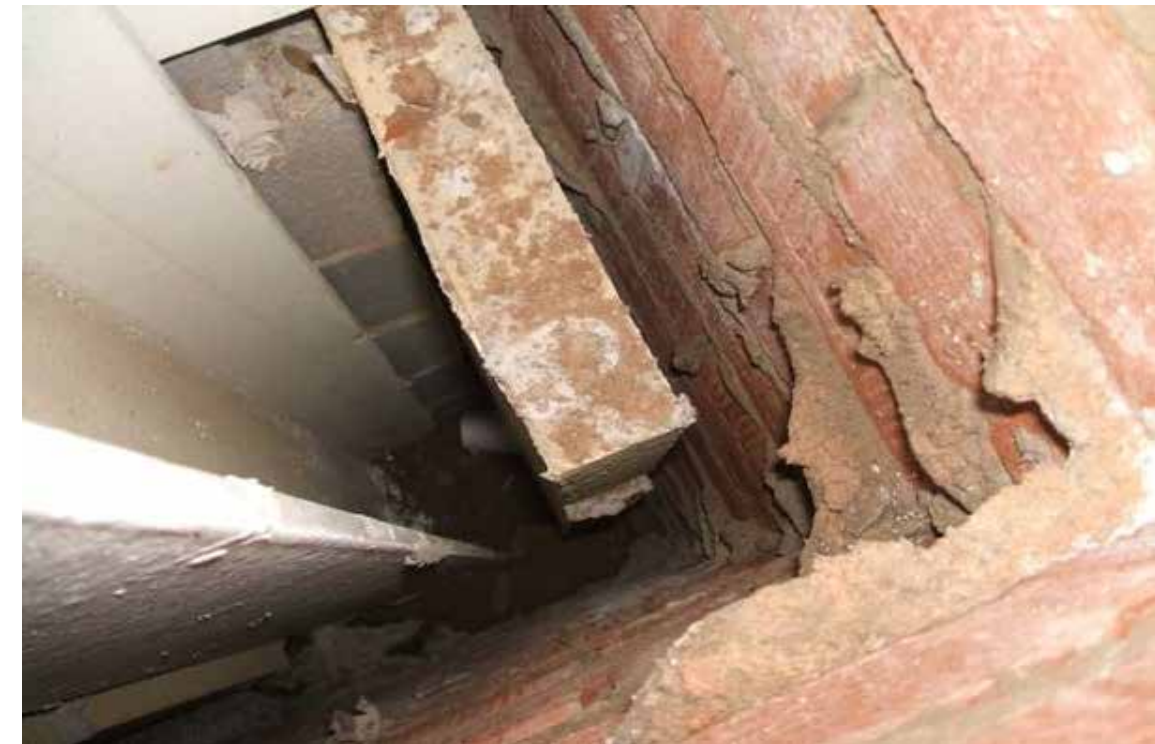
NOV 2011 PHOTOGRAPHS – NO VISIBLE EVIDENCE OF WALL TIES
