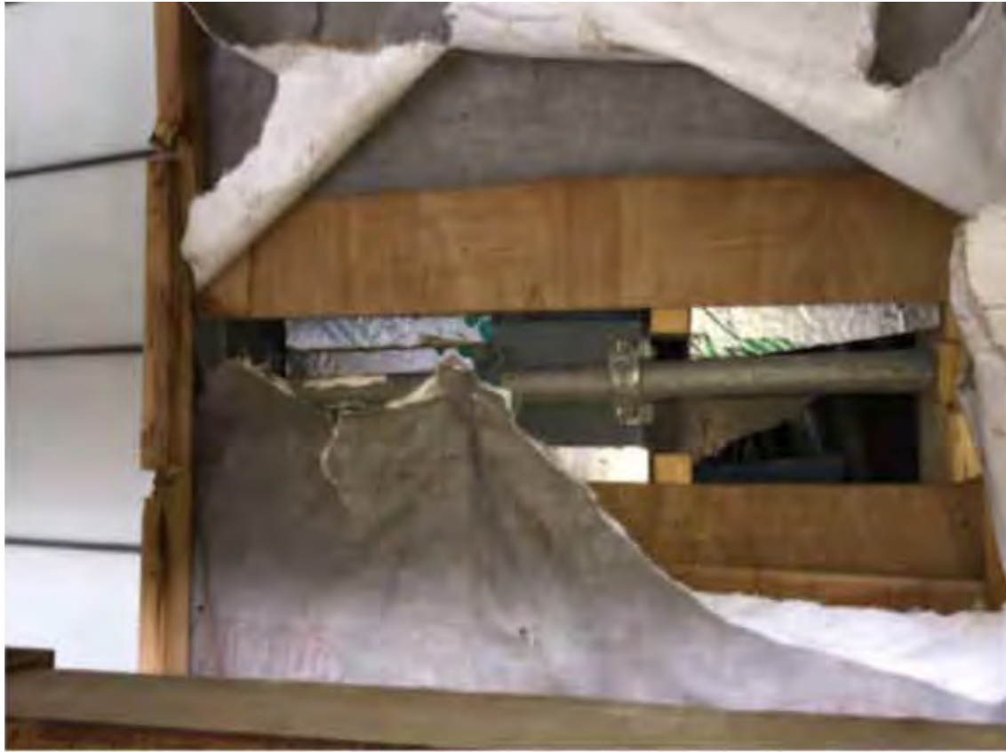
Scaffold tube remaining from original construction revealed on removal of external cedar cladding. Timbers and insulation bled around scaffold tube.
