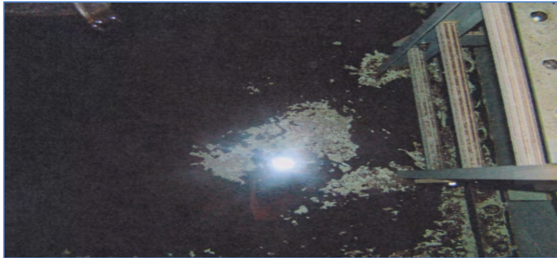
“The cold-water tanks show signs of organic matter and should be cleaned at the earliest opportunity and the system sampled for bacteria”. H&K 2011
