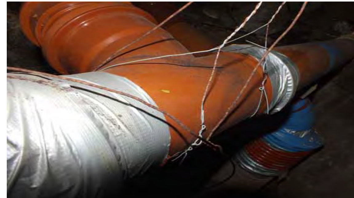
An example of the condition of underfloor drainage found
