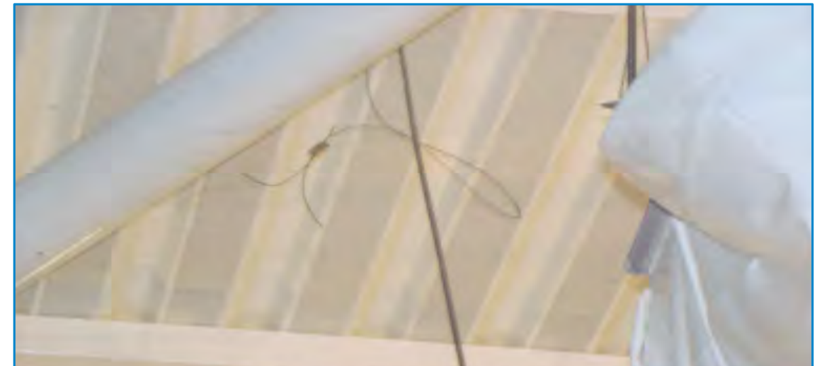
“Example of a snapped hanger to the pool ventilation duct work”. H&K 2011
