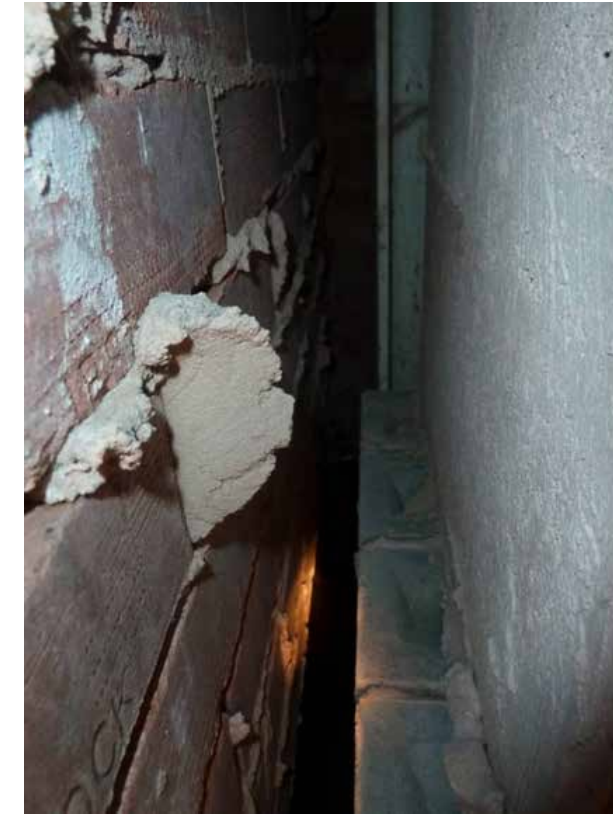
NOV 2011 PHOTOGRAPHS – NO VISIBLE EVIDENCE OF WALL TIES
