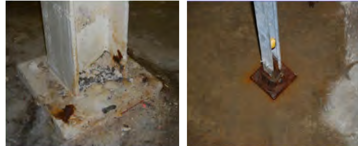
3. Corrosion of steel columns in the basement plant room
