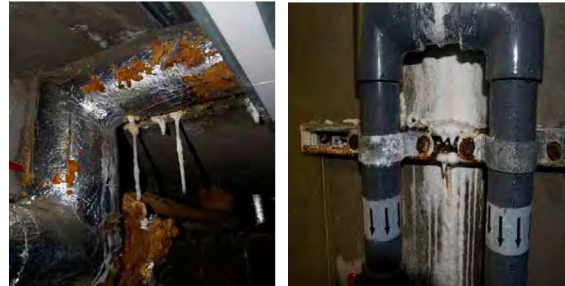
Examples of damage to pipe insulation and to galvanised fittings
