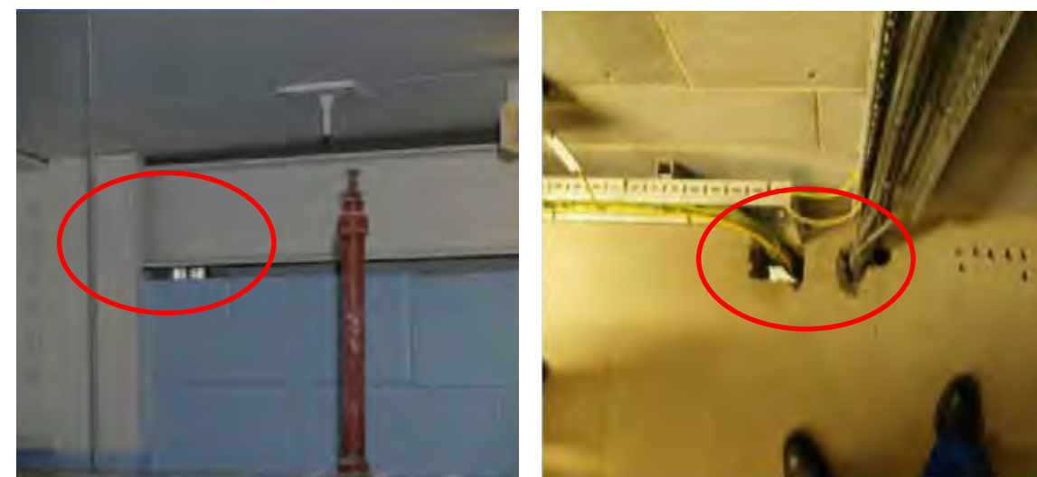
5. Two examples of many major omissions of essential fire-stopping, one in an escape corridor and second in the floor slab of a first-floor plant room
