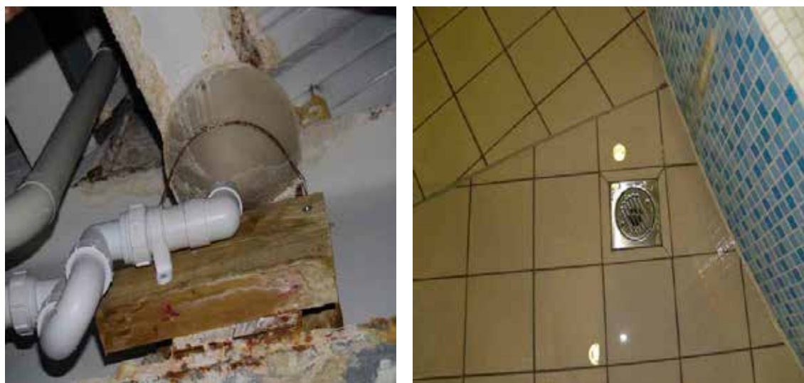
2. Domestic funnel collecting leaks from the spa pool and area of ponding at Spa
