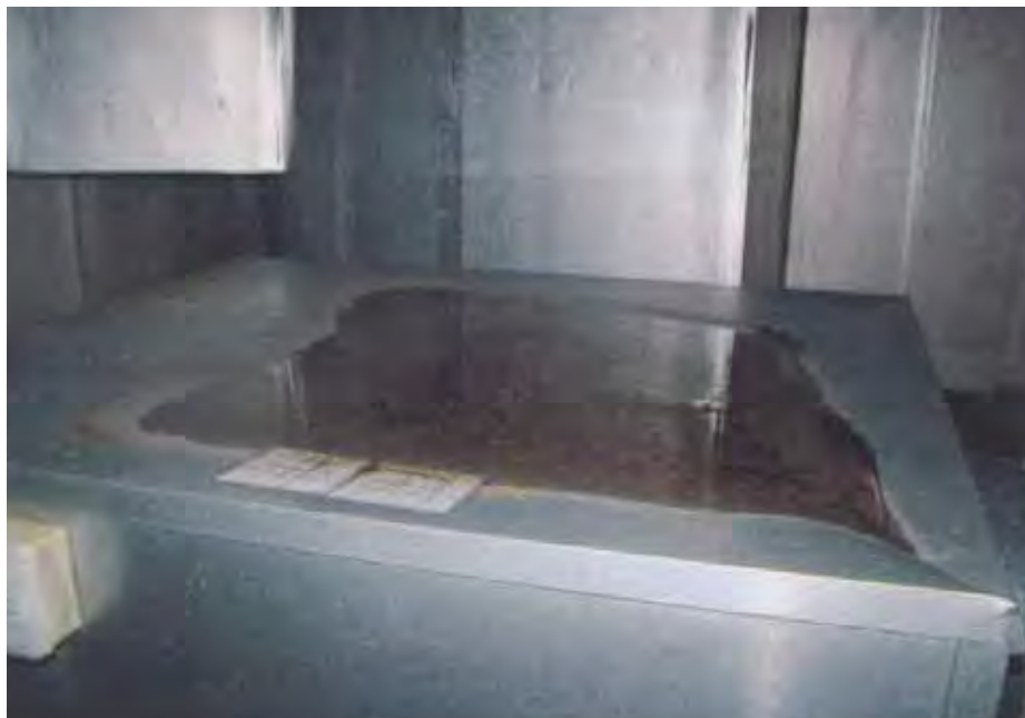
"Damaged extract fan cover allowing water to pond". H&K 2011
