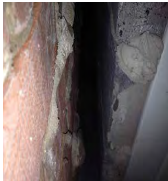
NOV 2011 PHOTOGRAPHS – NO VISIBLE EVIDENCE OF WALL TIES
