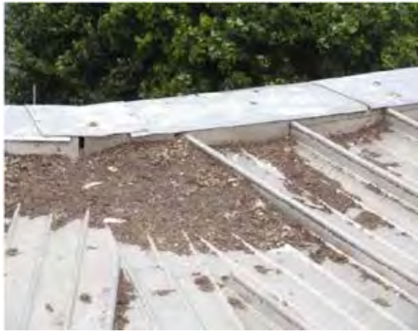
Build up of debris on roof and poorly fitted flashing
