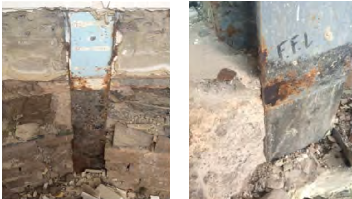
Corroded underfloor sections of steel columns
