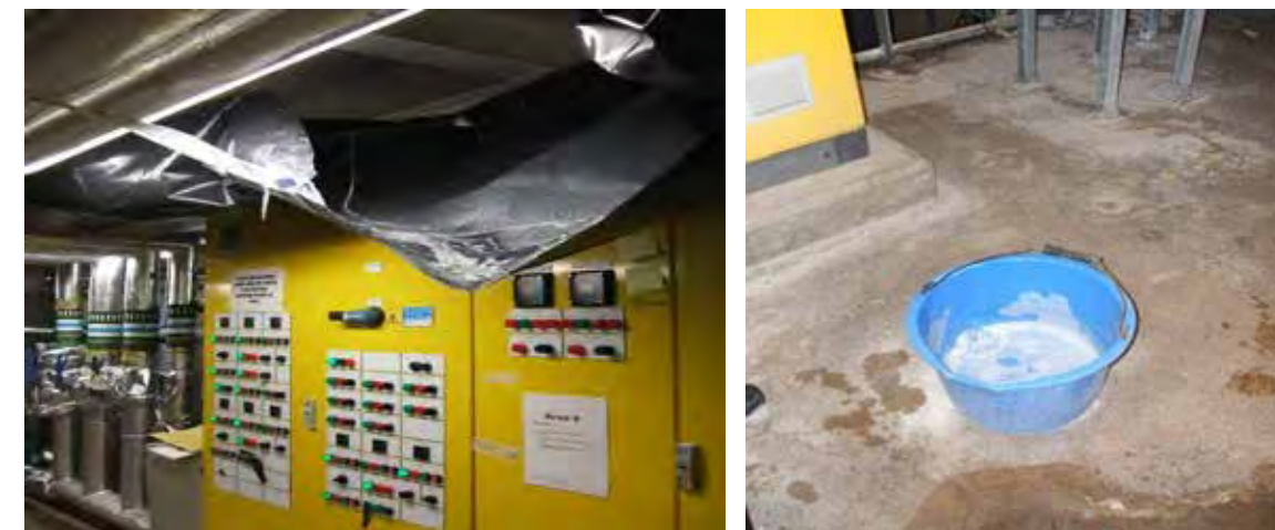
Polythene sheeting protecting electrical switchgear in the Plant Room from overhead water leakage, the redirected water being collected in a bucket.
