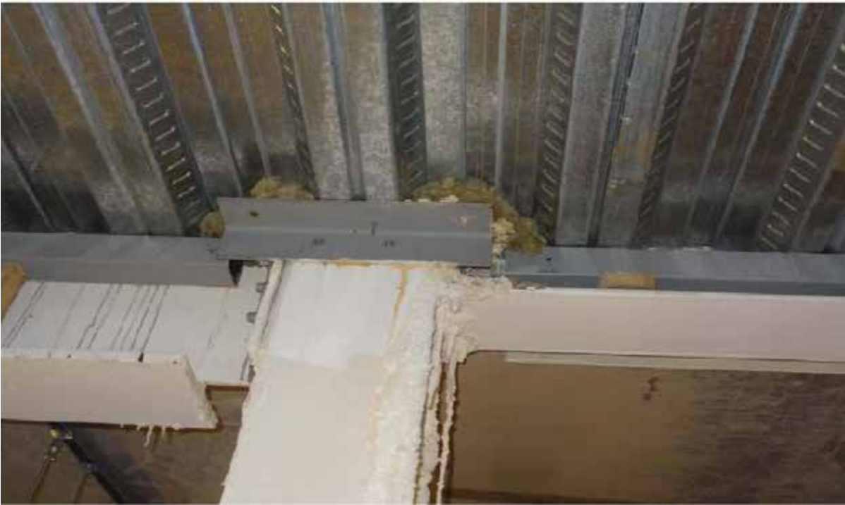
Leaks and lack of fire stopping
