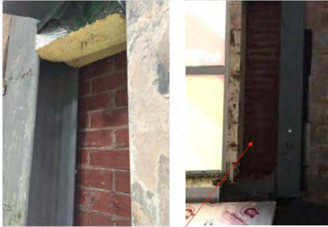
Piers 12. No inner leaf blockwork between Kalwall glazing and column. External brickwork has no tie back. Insulation boded.
