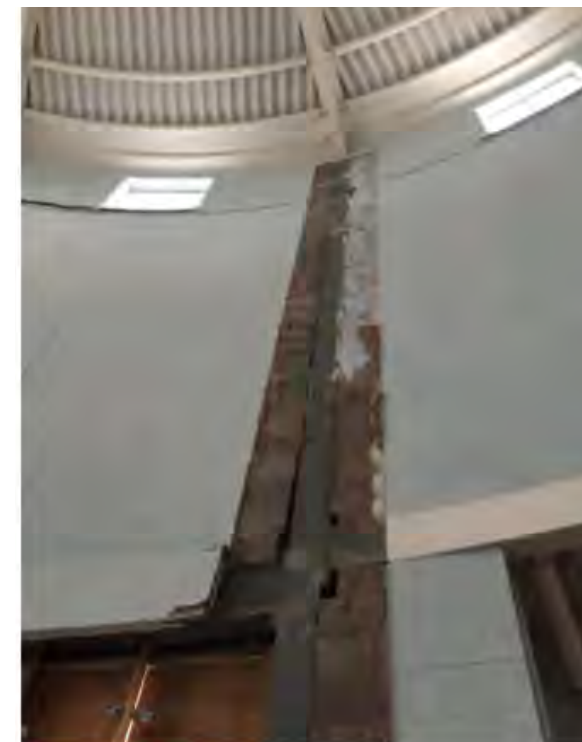
Piers 2. Block encasement removed. No ties in bottom 10 joint to left sides. No ties at all in right hand return. No ties to RHS of column in top section
