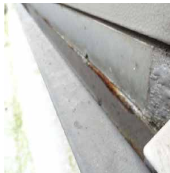
Corrosion to roof mounted plant
