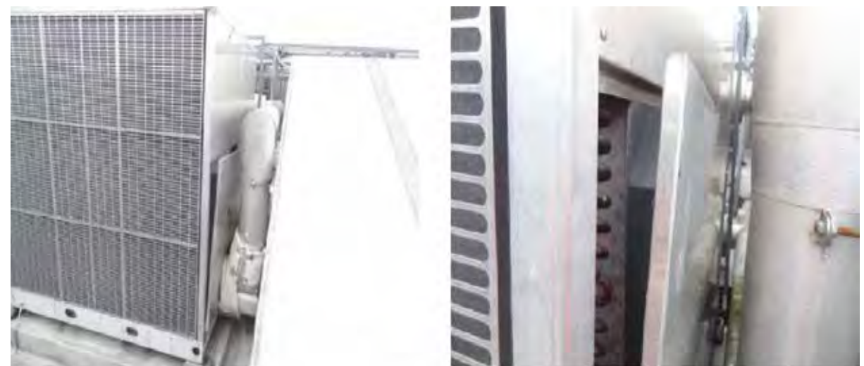
Unsecured and difficult to access panel on chiller
