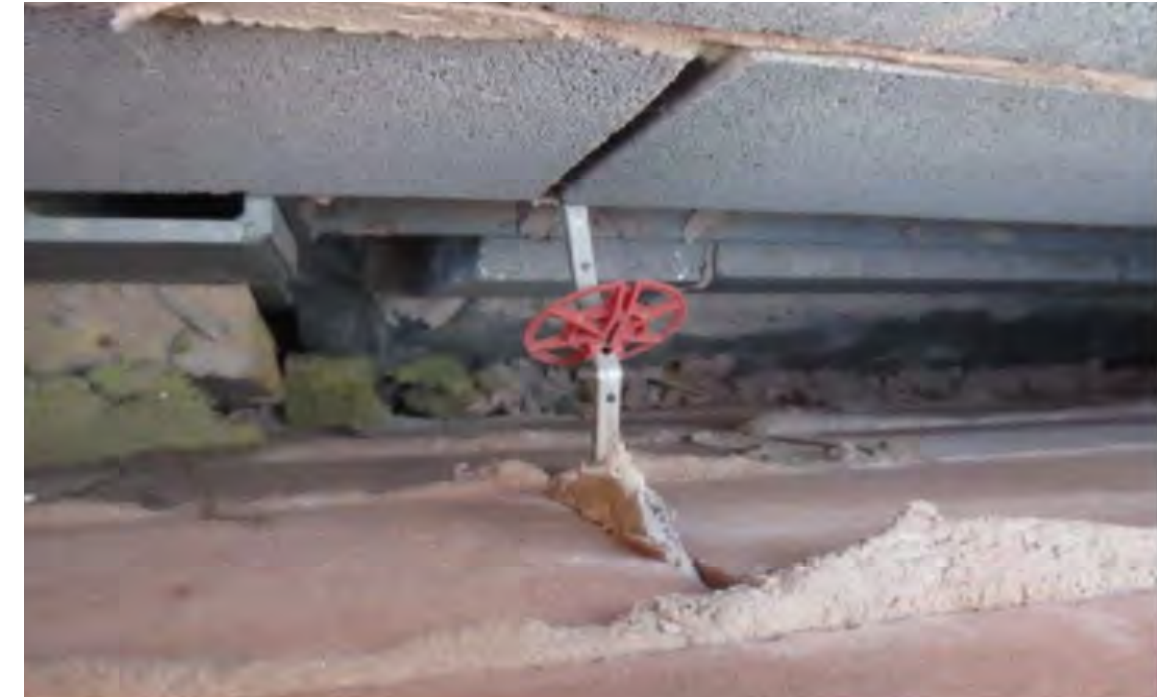
Bent wall tie, missing insulation and unfilled perpend joint.
