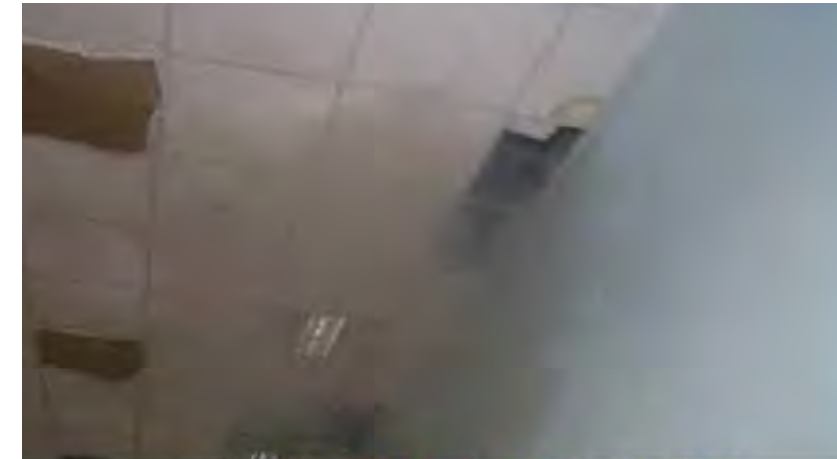
Test smoke pouring into dance studio from Wet area of building
