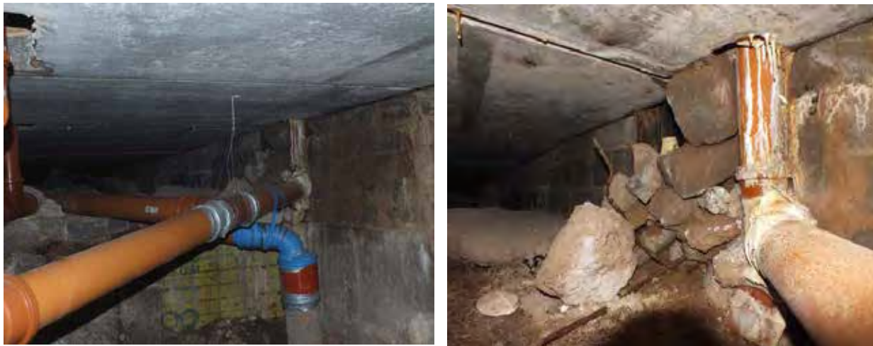
Examples of photographs of inadequately joined, supported and sealed drainage in the voids under DG One
