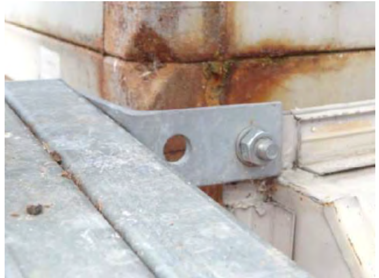
Corrosion to panels on roof
