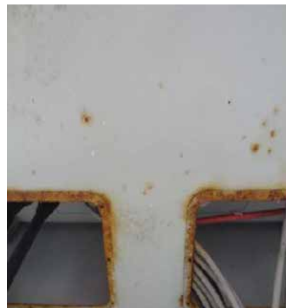
Corrosion to roof mounted plant
