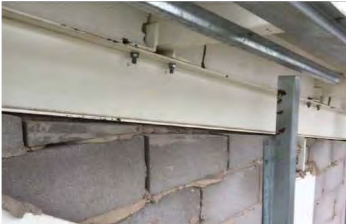
South Wall Main Pool. No supports to head of blockwork. Inadequate supports for external cladding panels.
