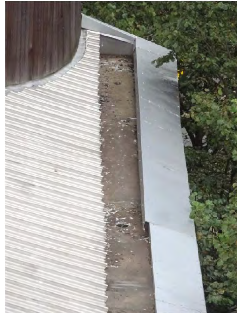
Poorly fitted and sealed flashing
