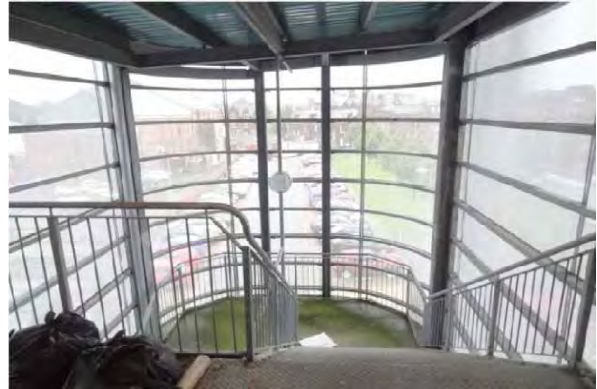
Staining and water ingress to escape stairs
