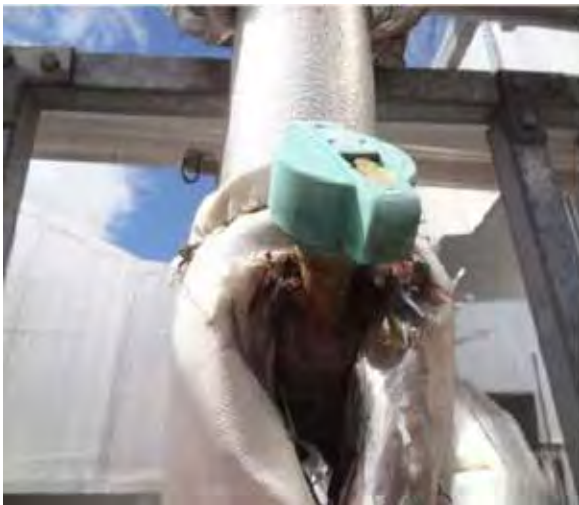
Corroding expansion chamber and valve
