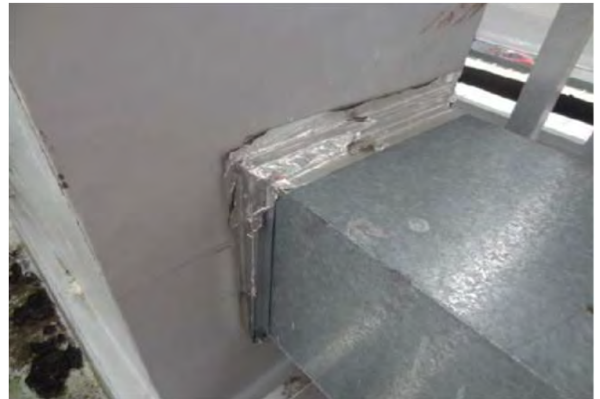
Poorly sealed ventilation duct
