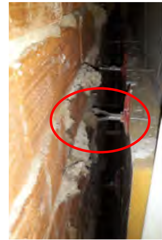
Quarter Landing 7. Ties too short. Insulation missing
