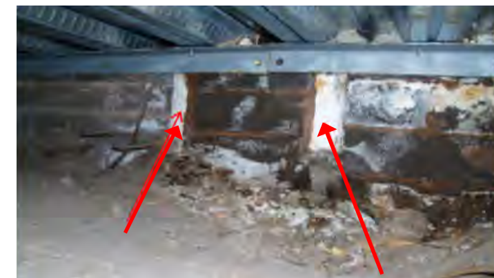
Steel columns indicated with red arrows are rusted and corroded
