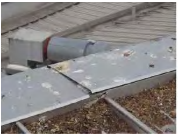
Build up of debris on roof and poorly fitted flashing
