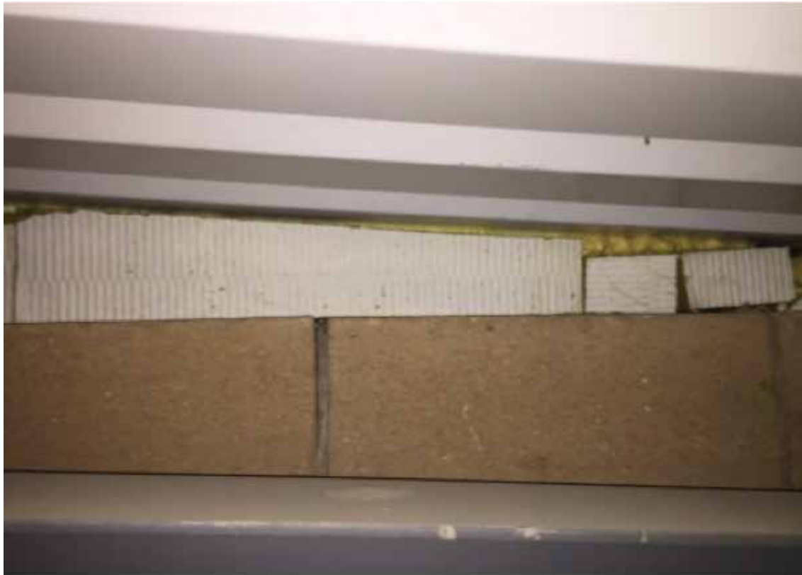
Wall to east of reception. No ties at wallhead
