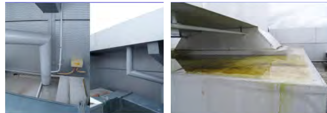
4. Examples of poor roof drainage. Water cascading from higher roof on to PVC membrane and ponding on roof due to no fall having been provided
