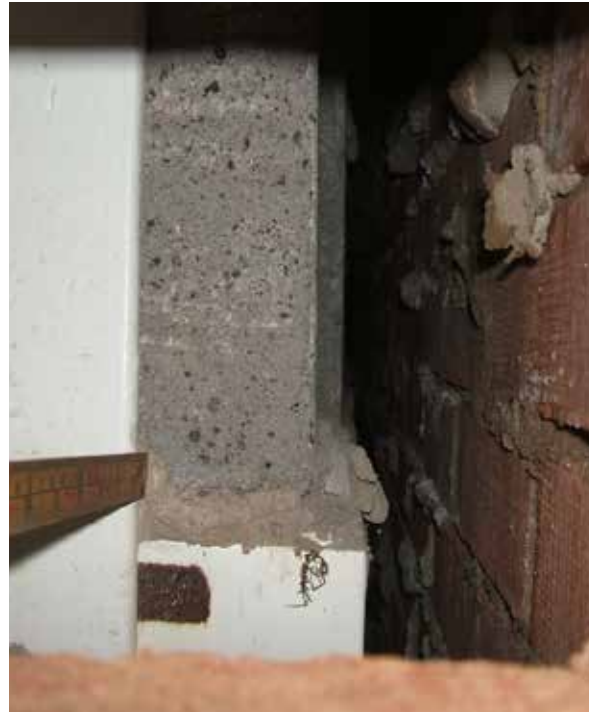
NOV 2011 PHOTOGRAPHS – NO VISIBLE EVIDENCE OF WALL TIES
