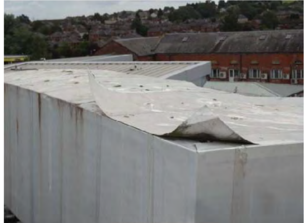
Potentially dangerous delaminating coverings
