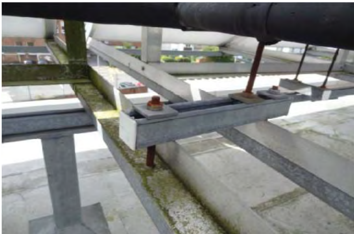
Corroded pipe supports
