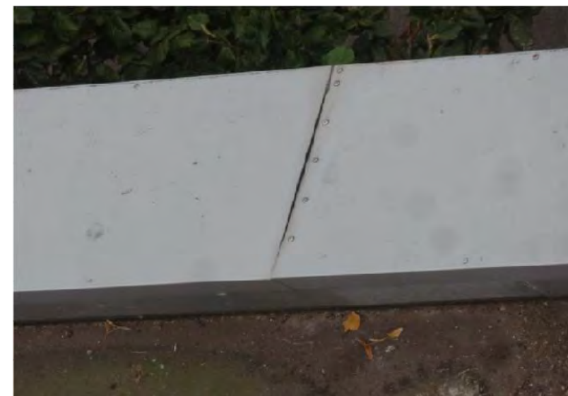
Poorly sealed and fitted coping flashing
