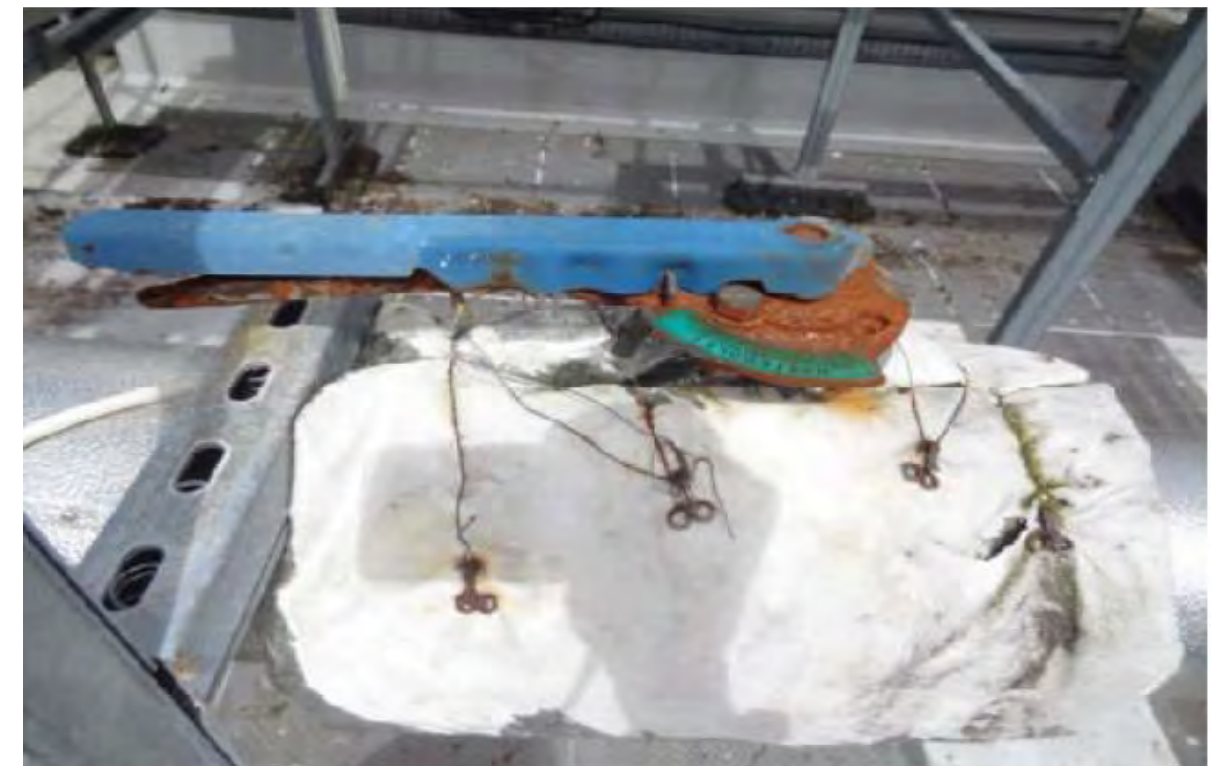
Corroded valve
