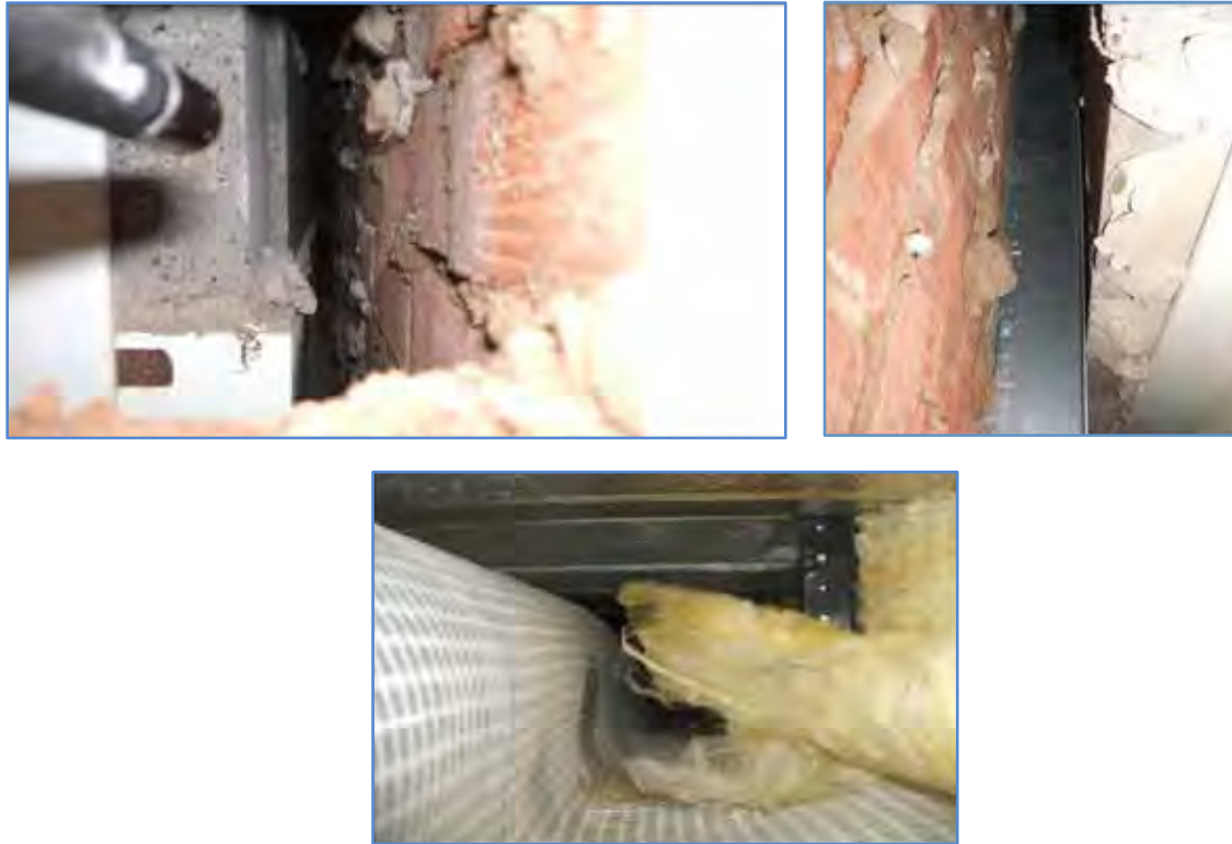
Absence or inadequate installation of insulation to walls and roof
