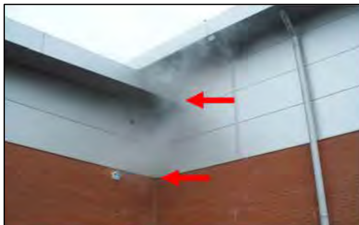
Test smoke rapidly escaping through eaves junction demonstrating lack of air-tightness
