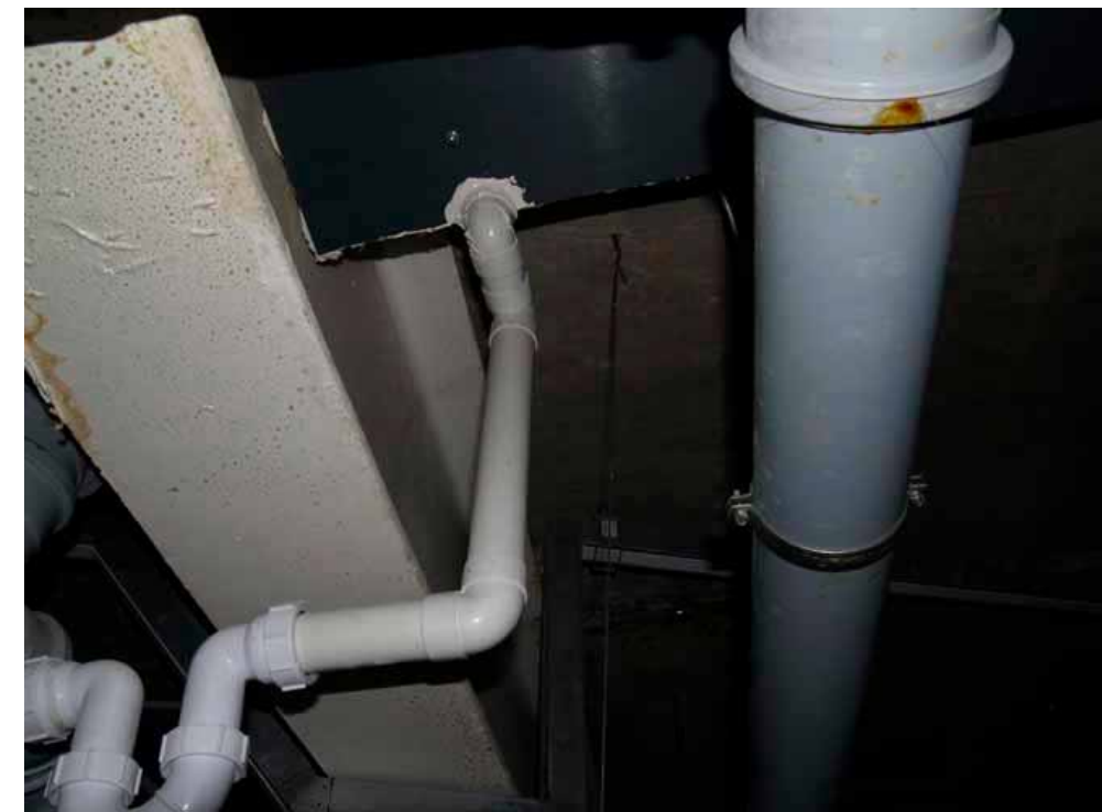
Leaks over changing areas and contractor's 'metal tray with drainpipe solution'
