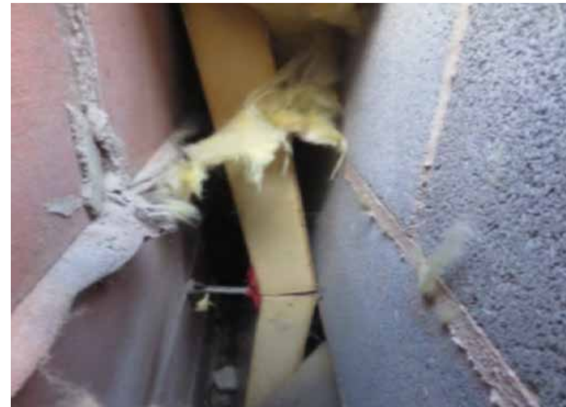
Improperly installed insulation
