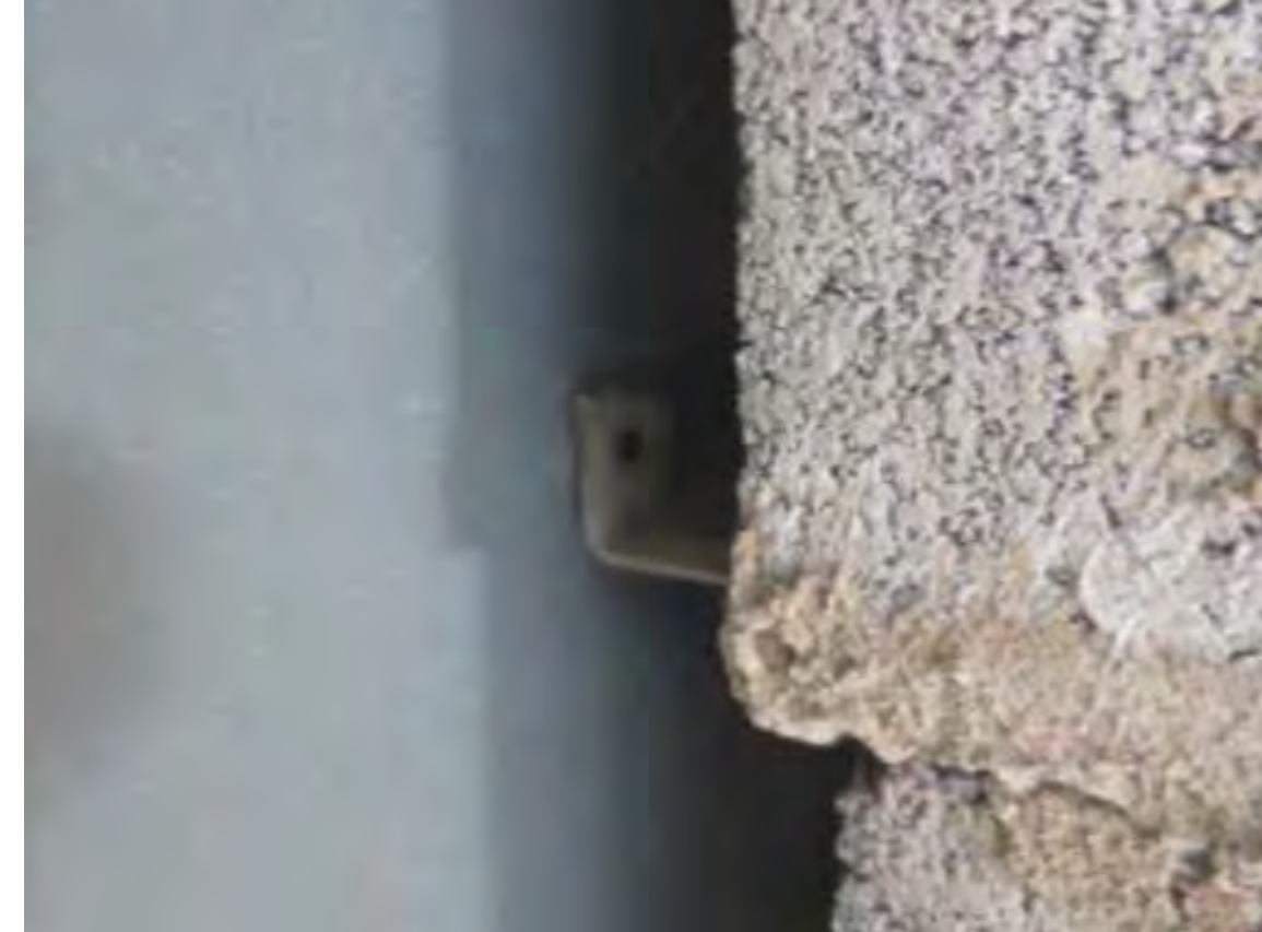
Exposed masonry. No shot fixing from tie to steel.
