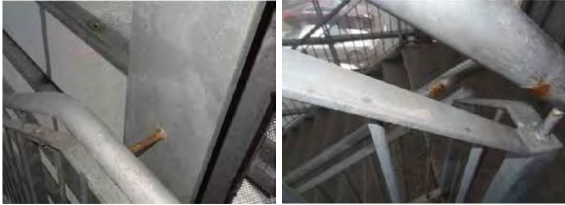
Corrosion to handrail support in escape stair.
