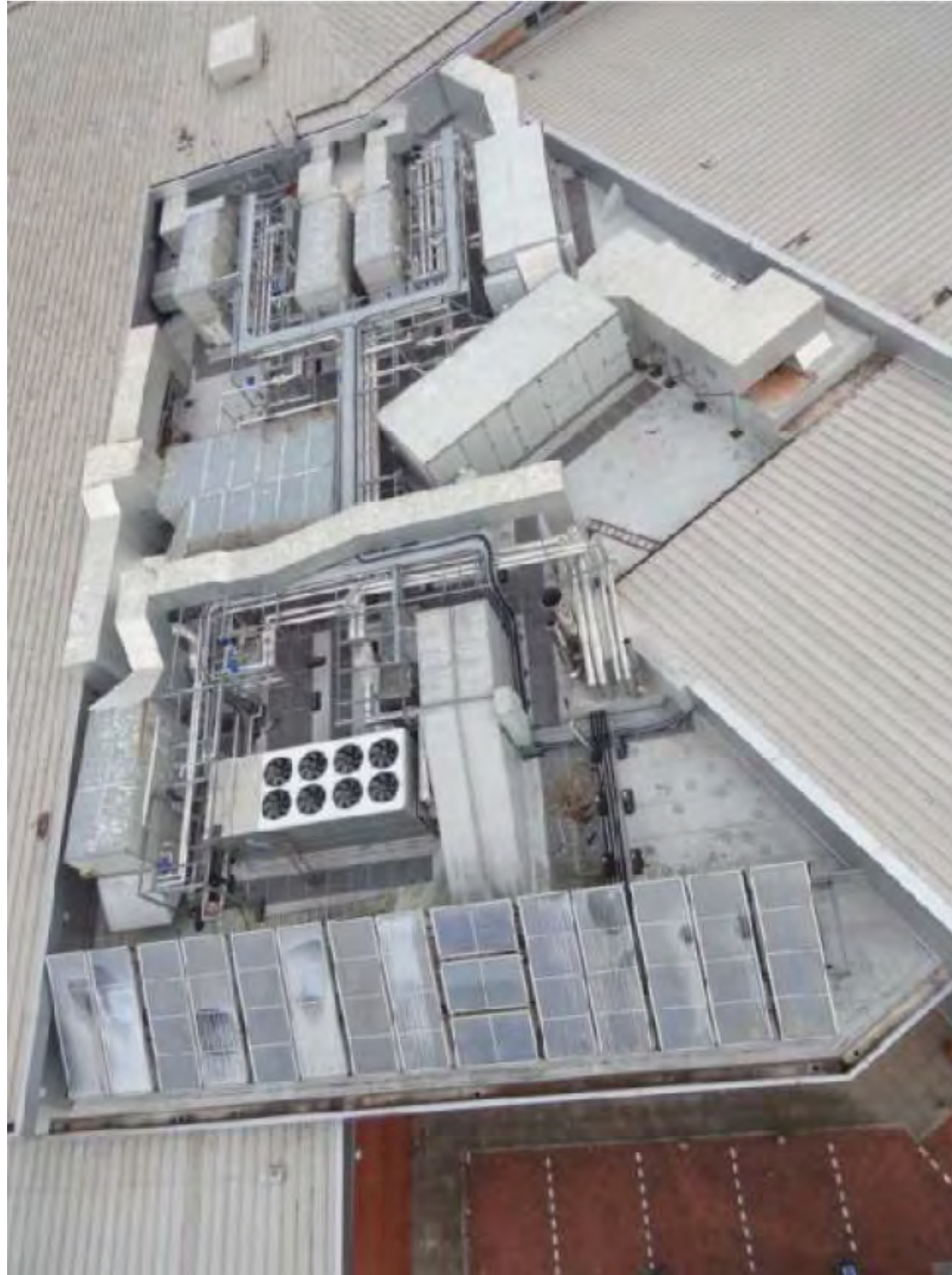
No proper maintenance access to plant. Poor condition of solar panels
