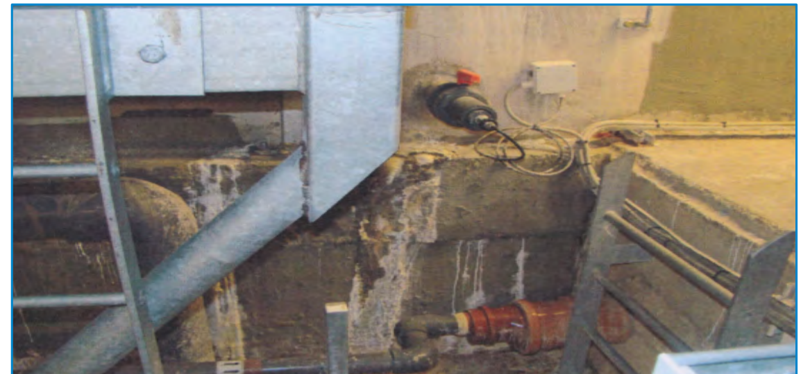
“Access to boilers for serving and replacement of tubes requires removal of plant. Also, evidence of water leaks from pool plant”. H&K 2011
