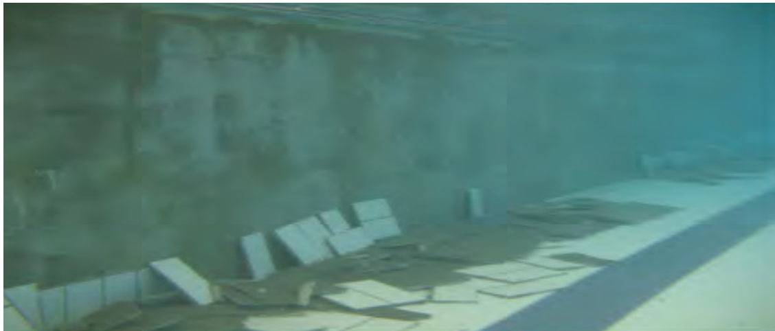
Tiles fully debonded from wall of main pool
