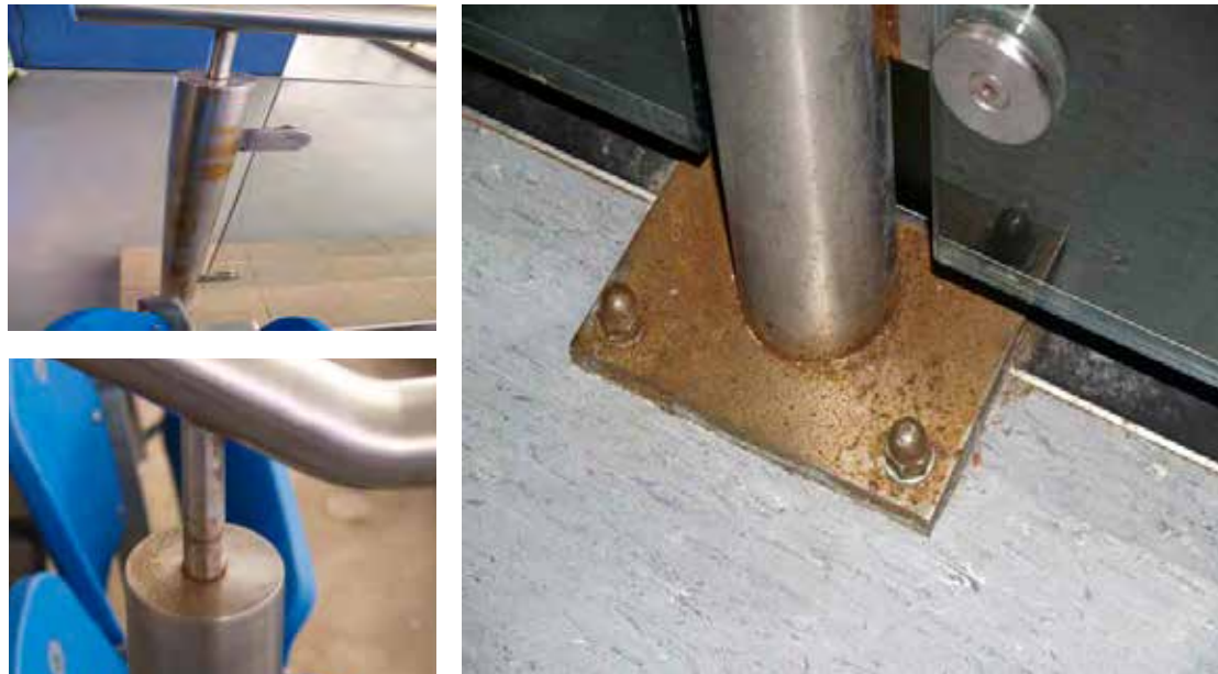
Examples of corrosion to steel fittings throughout the wet area
