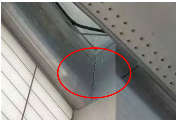
Photographs taken in Nov 2013 of cracking to blockwork encasement of columns in the Rotunda
