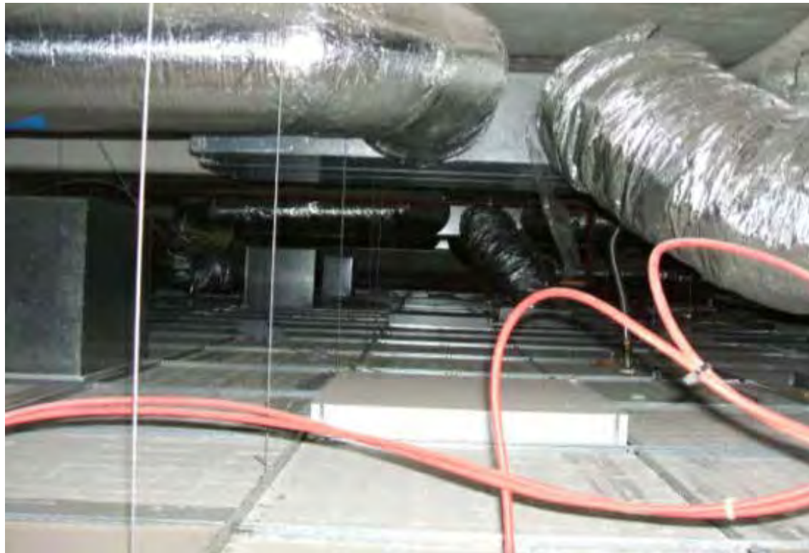
Luminaires without independent support resting on ceiling over gym
