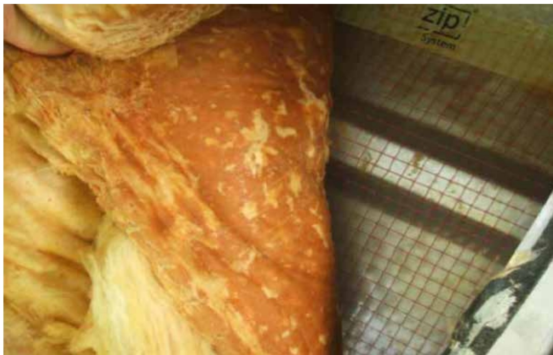
Insulation saturated with water at roof edge
