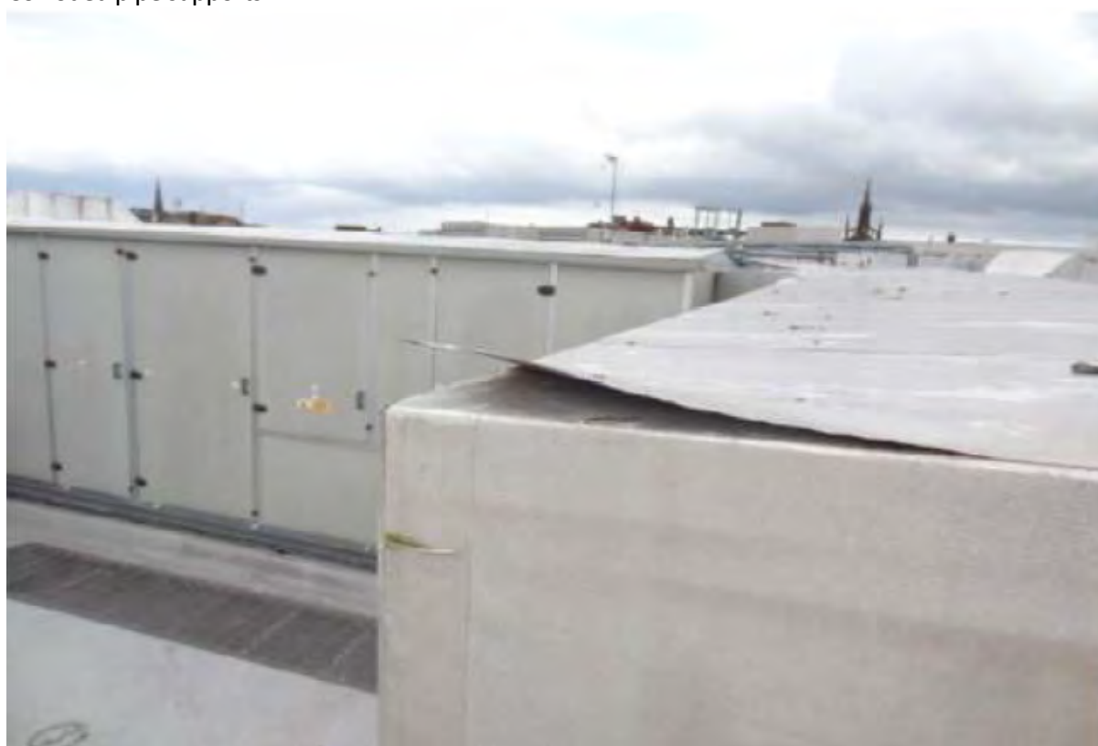
Damaged ductwork
