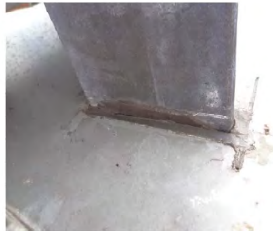
Poorly sealed penetrations through roof
