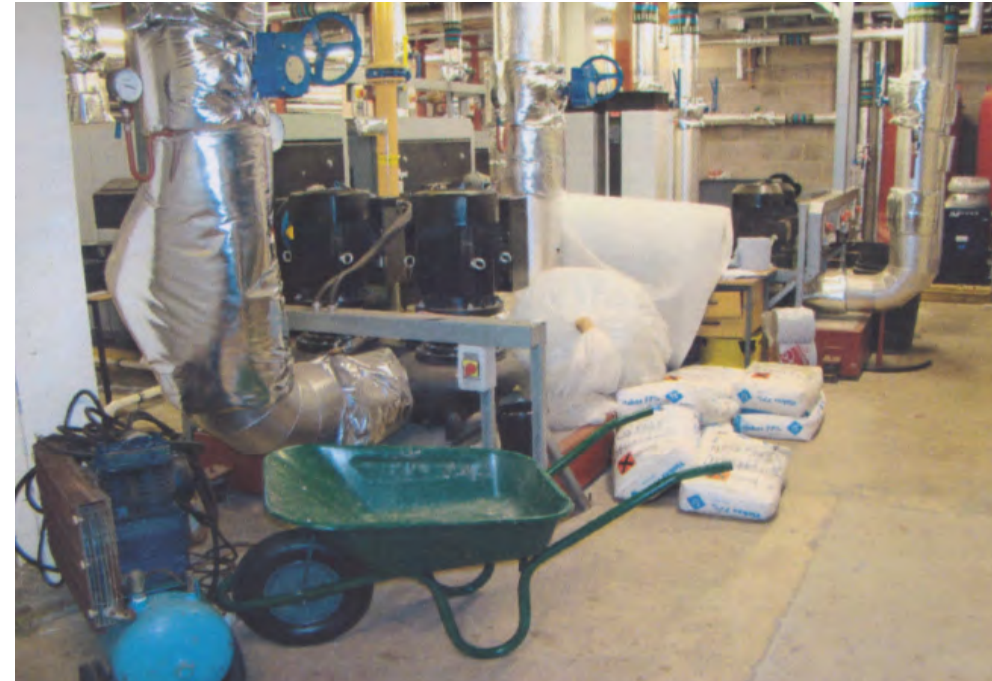
"Plant rooms are not presented in a manner that suggests regular expert attention is provided." H&K 2011
