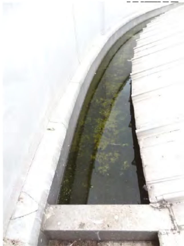
Blocked gutter at Rotunda
