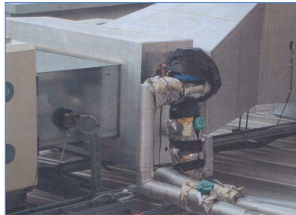
"Temporary repair to valve insulation" H&K 2011
