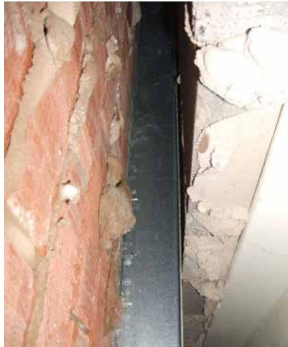
NOV 2011 PHOTOGRAPHS – NO VISIBLE EVIDENCE OF WALL TIES
