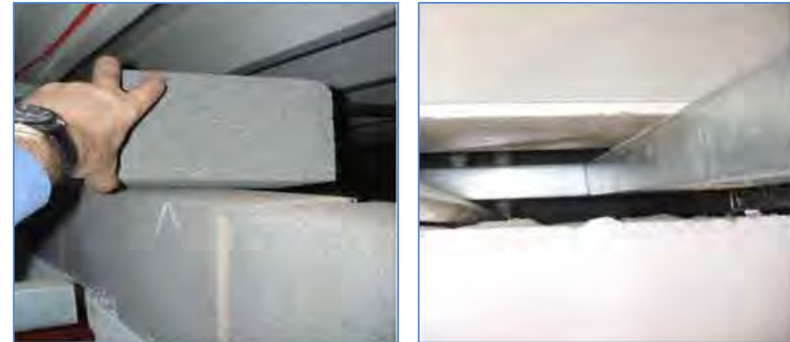
Defective fire compartmentation
