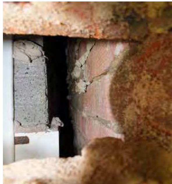
NOV 2011 PHOTOGRAPHS – NO VISIBLE EVIDENCE OF WALL TIES
