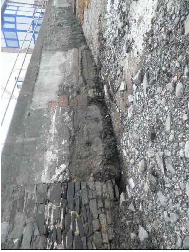
Plate 23: Detail of Breastworks wall deterioration.
