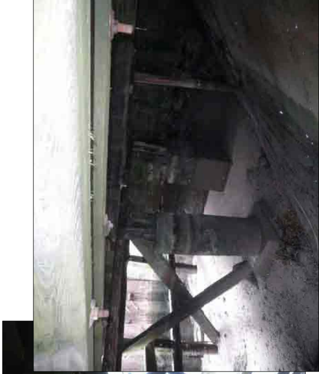
Plate 10: Under detail of West Pier showing breakwater construction.
