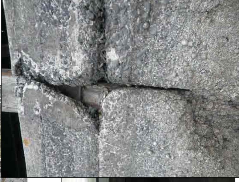
Plate 12: Deterioration of West Pier breakwater.
