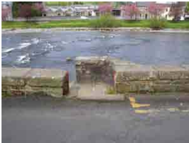
Figure 6.8 Unsealed Drainage Outlet at George Street
