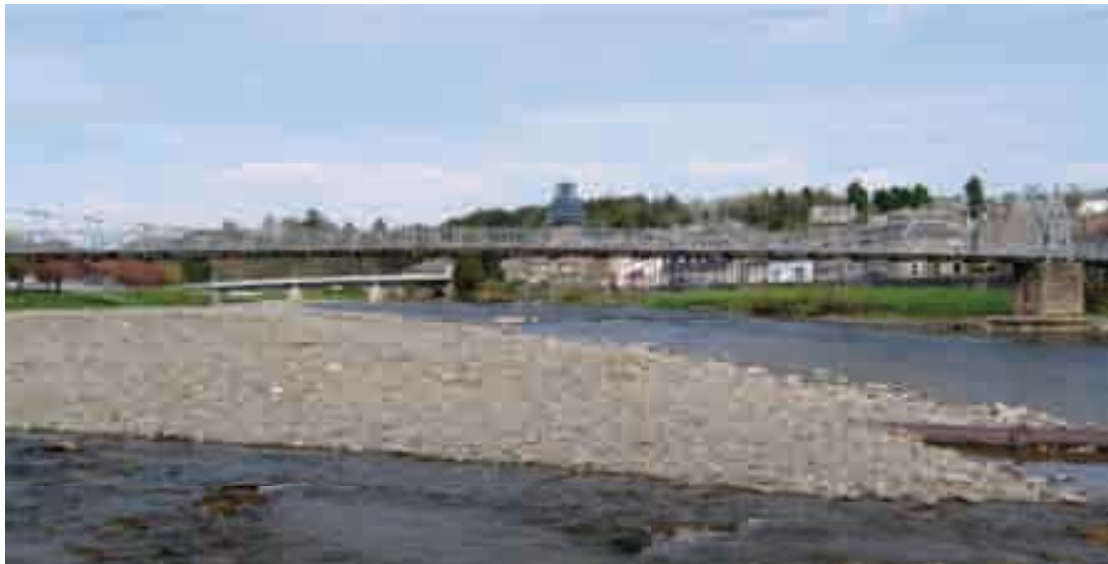
Figure 7.1: Gravel bar, looking upstream
