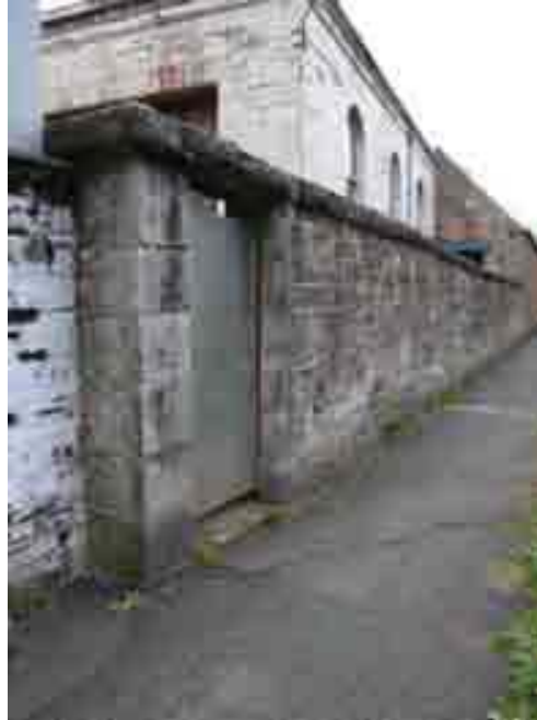
Figure 6.4 Pedestrian Gate at Mill (Note Gap below door)
