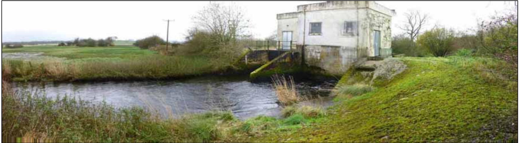
Plate 13 – Downstream side of Blackparks Pump station (pumps currently in action).
