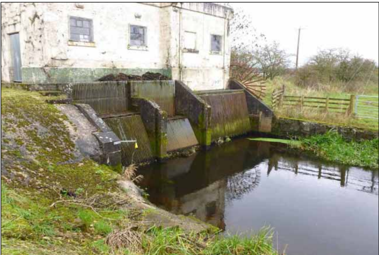
Plate 19 – View of upstream side of pump station.
