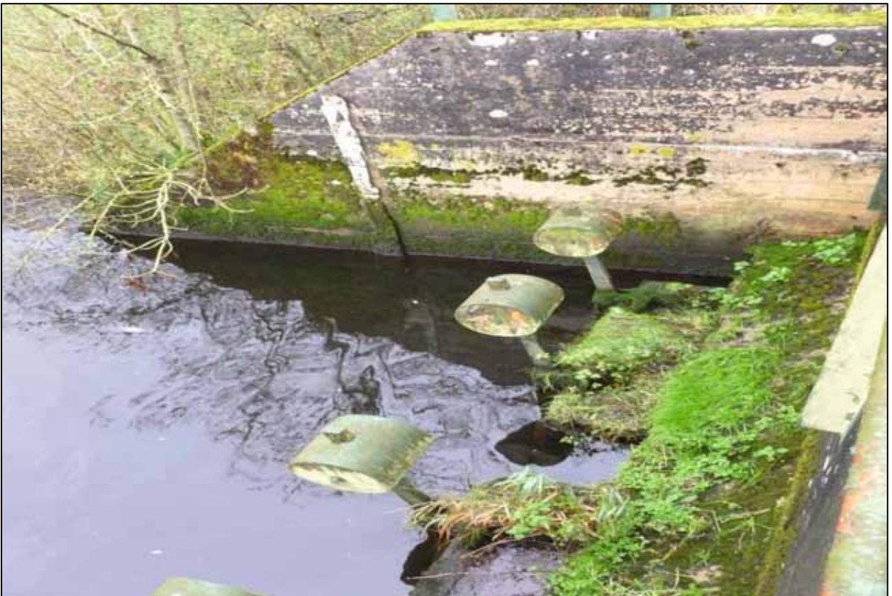
Plate 17 – View of non-return culvert gates at Blackparks Pump station.
