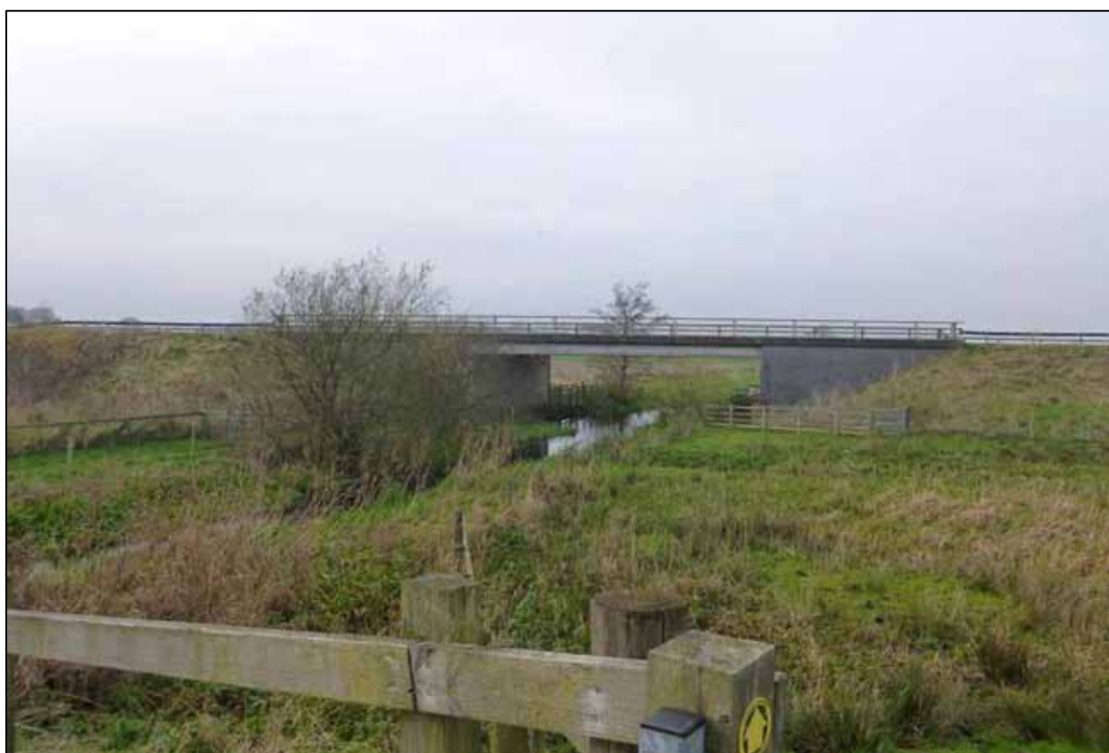
Plate 15 – View of upstream side of A75 road bridge.
