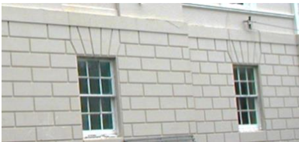
Stucco elevations, Dumfries
