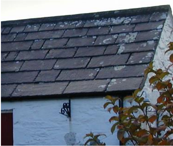
Graded Lancashire slate roof
