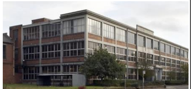
Early 20 th century former car factory, Heathhall, Dumfries
