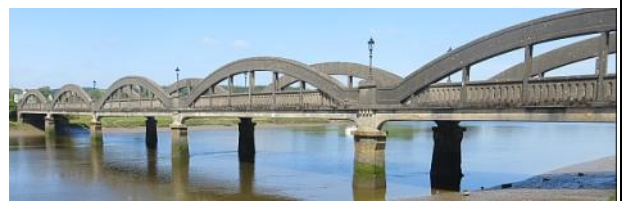
Early 20 th century reinforced concrete and steel bridge, Kirkcudbright
