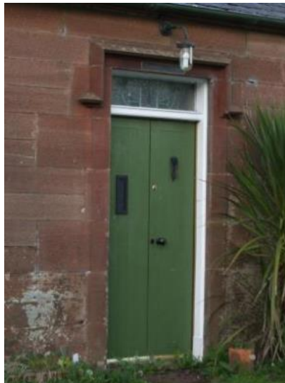
Patterns of slatework found in region. Sandstone drip moulds over gate lodge door; unusual corbelling detail on corner of sandstone house.
