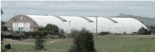
Former plane hangar at Heathhall
