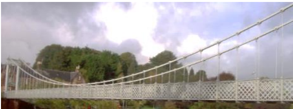
19 th century suspension bridge, Dumfries
