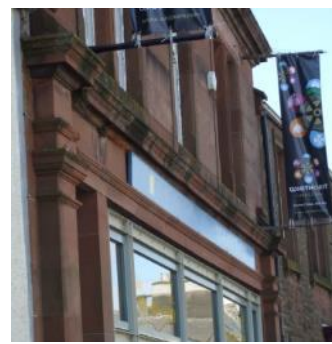
Early 20 th century commercial building in Whithorn, which differs from its neighbours due to use of ashlar sandstone and classical details
