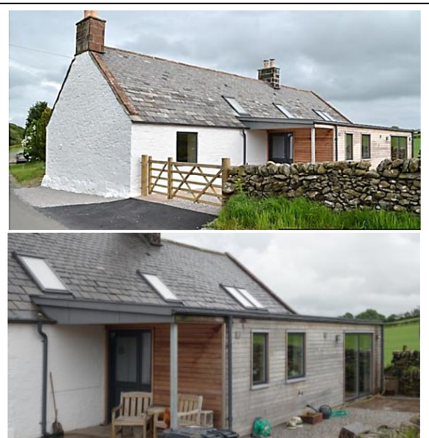
Dumfries and Galloway Design Awards, 2016 winner in the category for work to existing buildings: Killylour, by Simon Winstanley Architects
