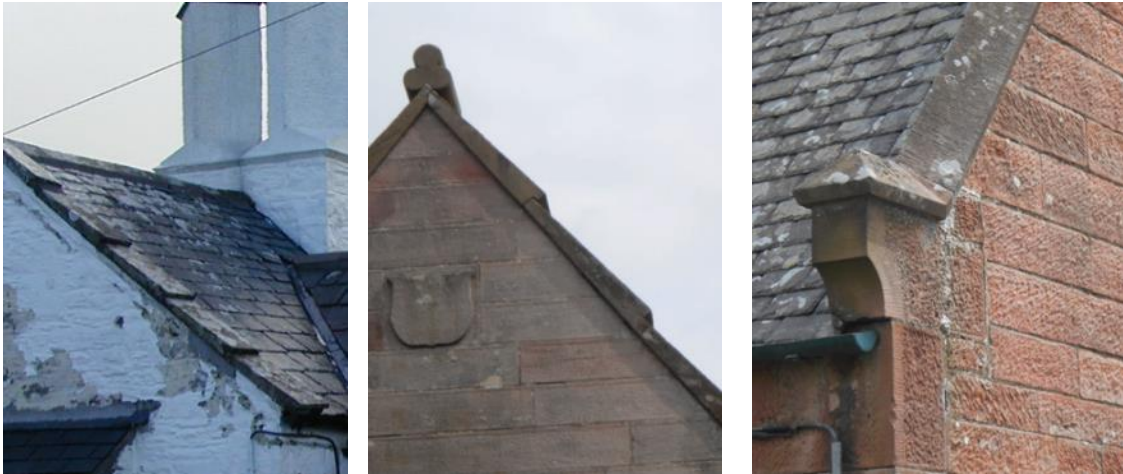
Examples of varied roof line details: a selection of skewstones – stepped, shaped, interlocking and plain; a shaped gable stack; and decorative skewputts and finial
