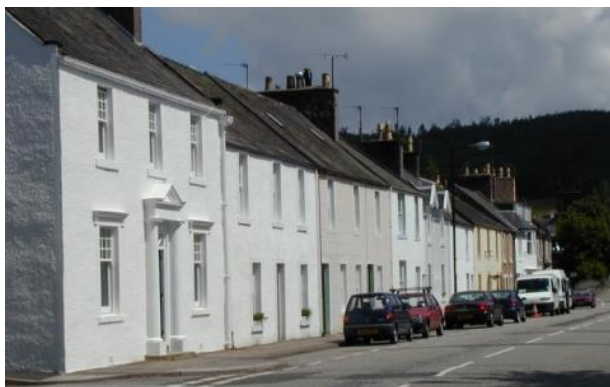
Gatehouse of Fleet Conservation Area: The forward building line is common in both streets; house widths are repeated but not uniform; and roof heights vary in both streets although none are more than 2 storeys. The social hierarchy is legible in the houses within the streets.
