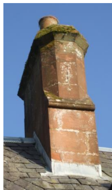
Both functional and decorative sandstone chimney: hexagonal shaped ashlar on a moulded haunch
