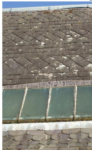
Lodge with overhanging slate roof, angle cut tiles and verge board; decorative slate work and example of 'double lap open tally' slating in Nithsdale.
