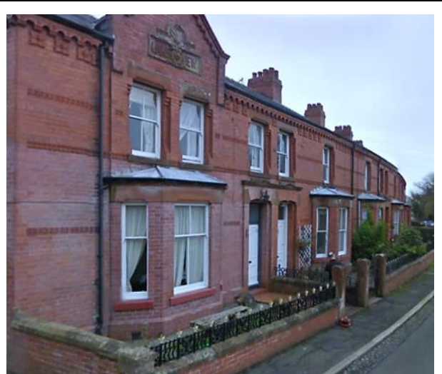
Lakeview Terrace, Powfoot - a continuous brick façade with string course and cornice; regular bay windows and chimneys and front facing gable 'end stops'.
