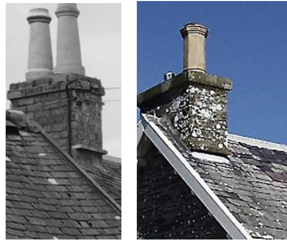
Chimneys with thackstones: evidence of earlier thatching
