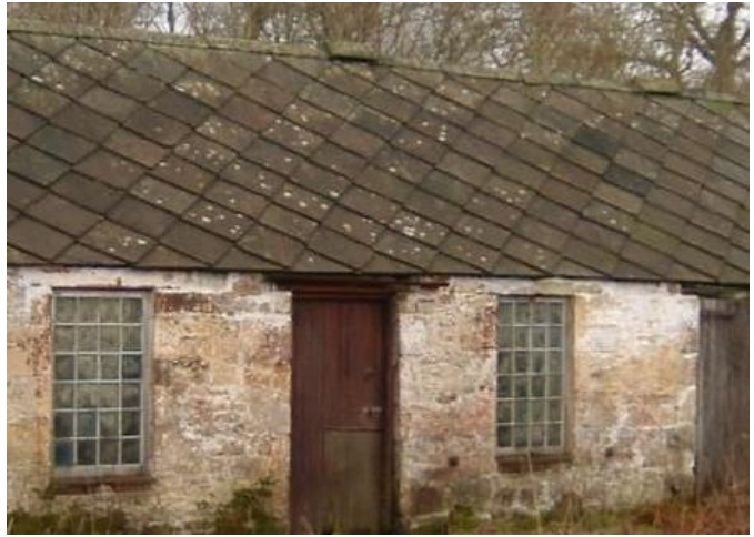
Sandstone flagged roof
