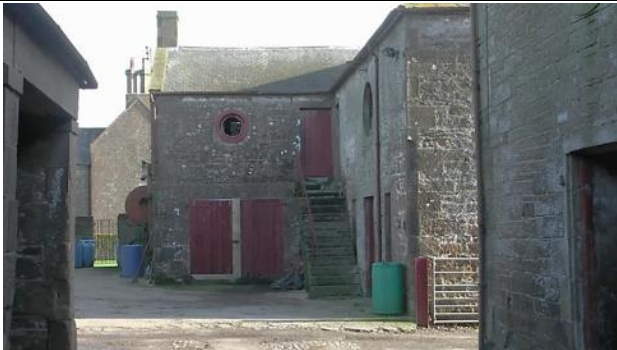
Spaces between traditional farm buildings relate to their original function and have historic significance
