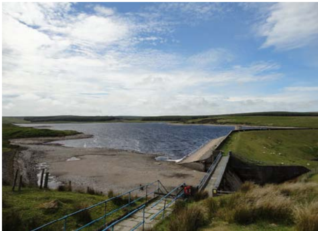
Reservoir infrastructure and forestry in parts of the Plateau Moorland
