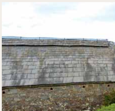
ventilators at ridge
