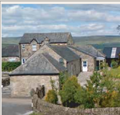
south east; dressed stone at corners & openings fieldstone - buff/honey brown
