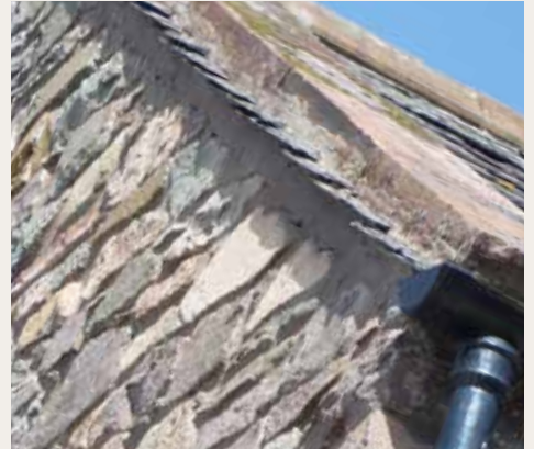
slates extend behind cope
