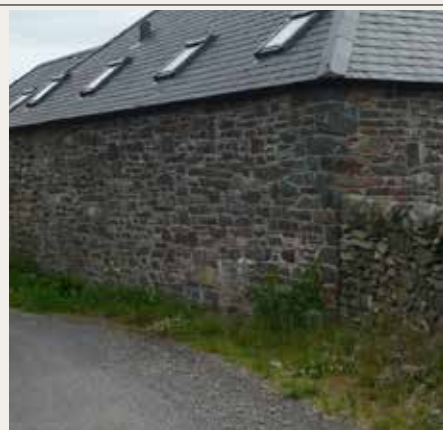
Kirkcudbrightshire; dark grey stone and light grey margins forms rubble wall, no ashlar or dressed stone at corners
