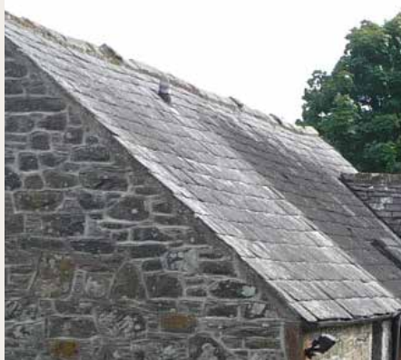
plain eaves & verge detail with no gutter
