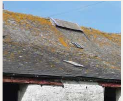
lichen on roof
