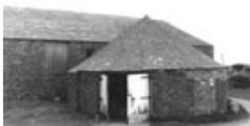
This has led to great variation in texture, thickness and colour. Many roofs are laid with the slates reducing in size towards the ridge. This grading should be retained. New roofs and repairs to existing roofs should follow local traditional finishes. New slates should be of the same type, or if these are unavailable, should be closely matched for thickness, colour and texture.
