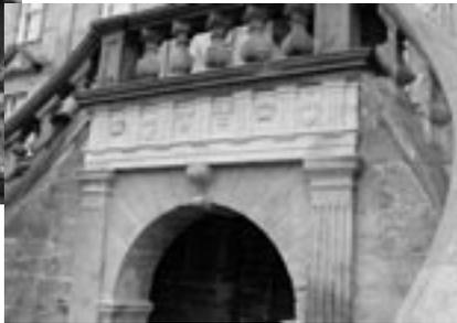
to facing stone. Replacement or dressing back should not be undertaken lightly. All new stone should be worked and tooled in the same manner as that is being replaced.
