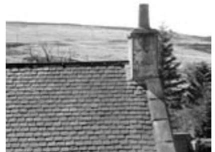
Skews should be kept and repaired in matching stone. They are an important part of the architecture of buildings and in terraced groups
