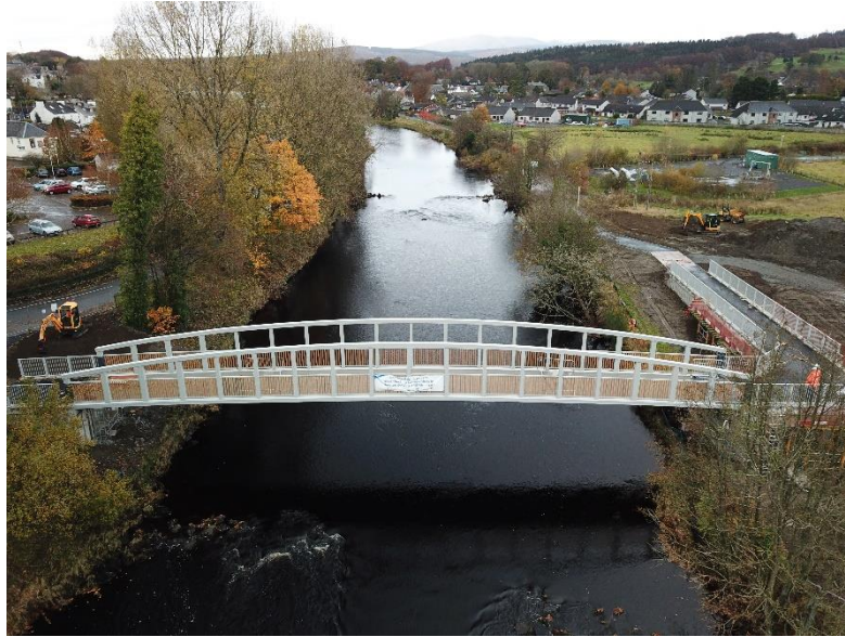
Bridge under construction
