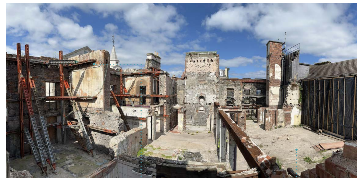
Internal view looking north
