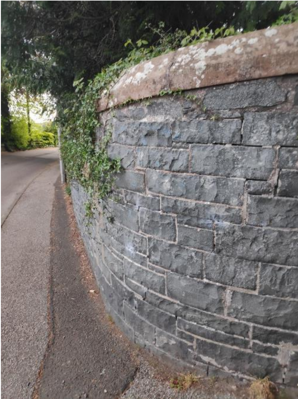
Figure 7: Whinstone is a plentiful stone locally; its use for building is sustainable and it supports the local landscape and townscape character.
