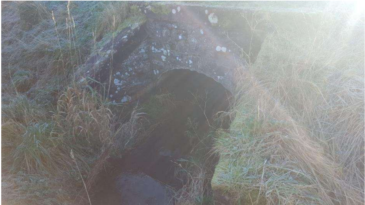
Photo 3: Crosslaw Burn culvert (upstream side)
