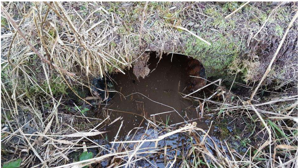
Photo 4: 0.6 m bypass culvert (upstream face)
