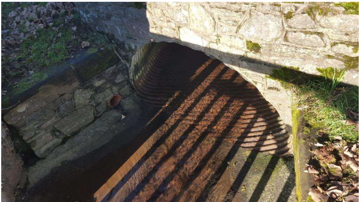
Photo 2: Crosslaw Burn culvert (downstream side)
