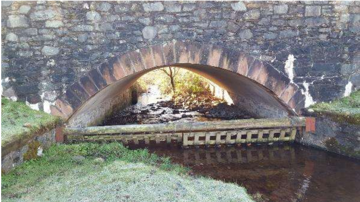
Photo 7: A708 road bridge over Frenchland Burn.
