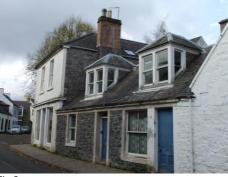
3. The widespread use of uPVC and aluminium windows, doors and other elements. Ahistoric building starts to lose its integrity and authenticity when any part of its original fabric is replaced. A large number of buildings throughout the conservation area have regrettably been the subject of window replacement using inappropriate and poor quality window units. (fig. 2, 7, 10, 12, 13)
