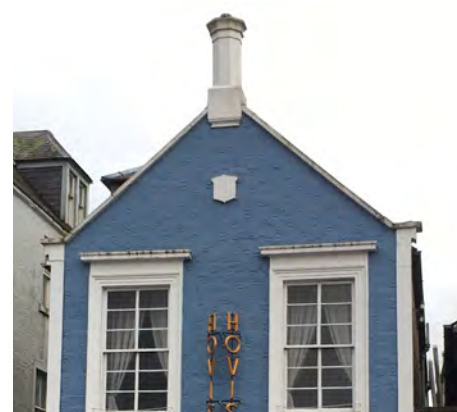
Octagonal chimney example
