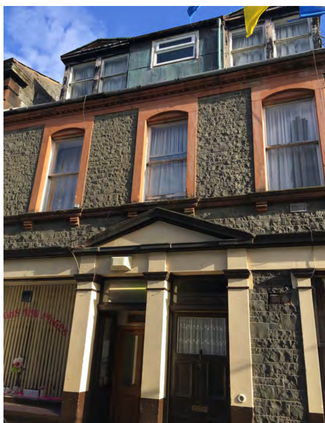
Building on Well Street
