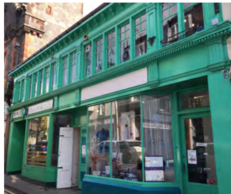
Shopfront on Well Street
