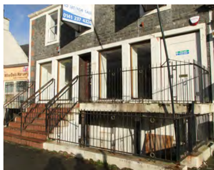
Derelict former 'Pringle' shop on High Street
