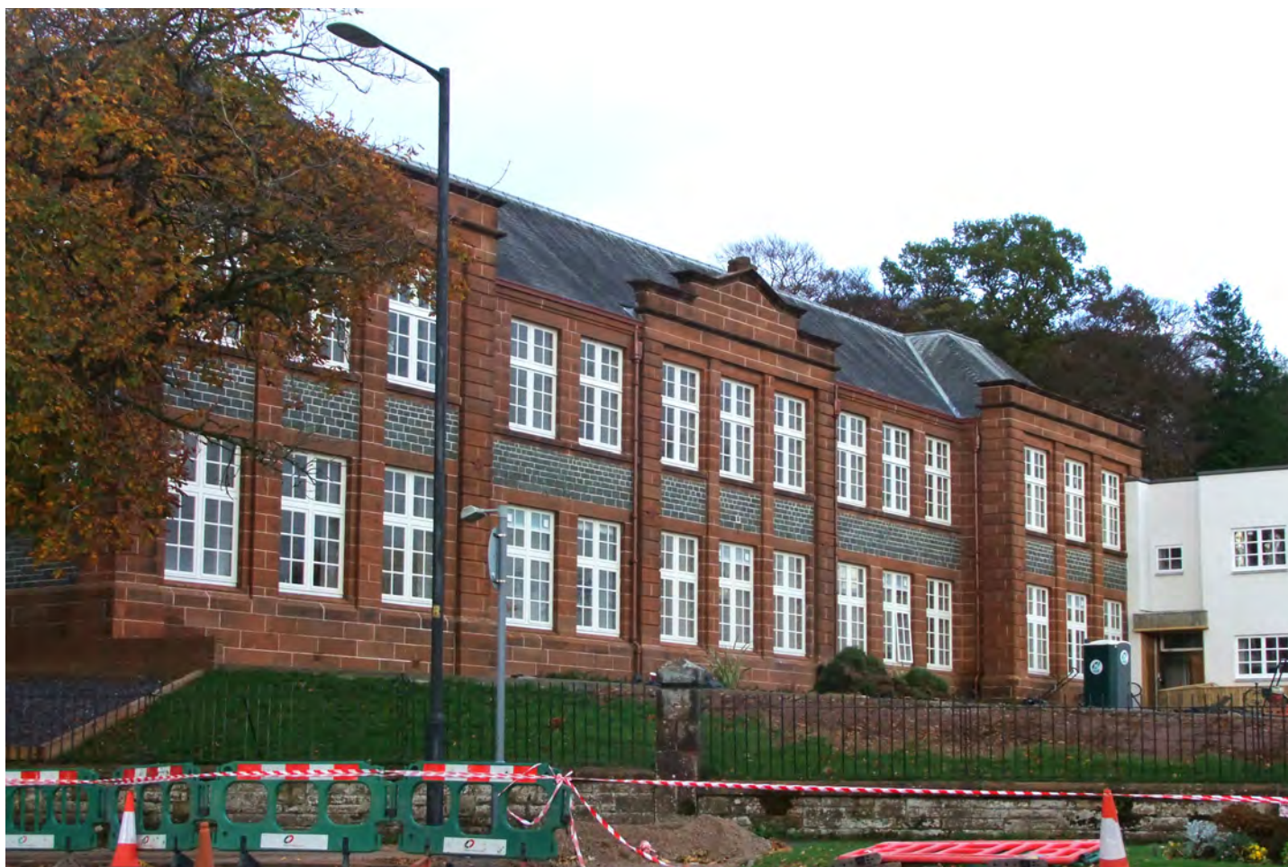
Moffat Academy, now converted to residential flats
