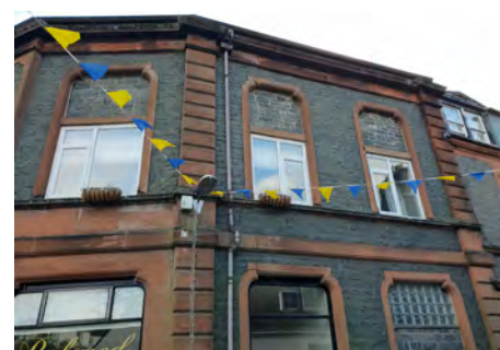
Building with whinstone laid in diminishing courses
