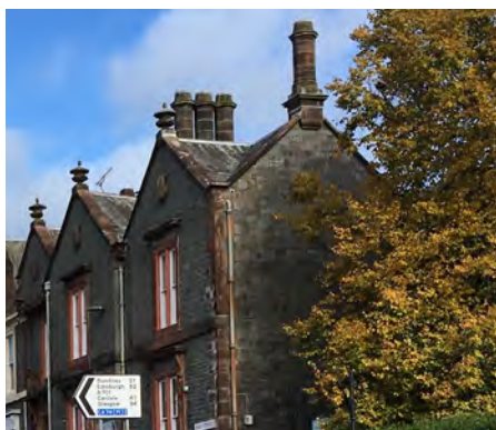
Octagonal chimney example
