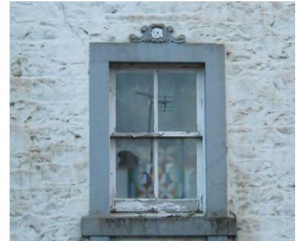
Finial detail on a building on High Street
