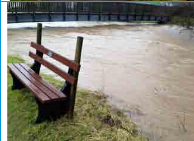
Flood level at footbridge. Estimated to be approximately 0.7m from bridge soffit.
