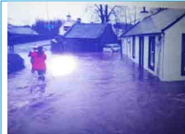
Flooding on Dunreggan Brae looking west towards High Street Bridge
