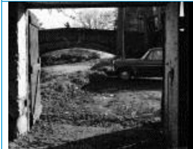
Presumed to be taken from the right bank of the Dalwhat Water looking downstream to the upstream face of the main road bridge (prior to the construction of the sheet pile wall).
