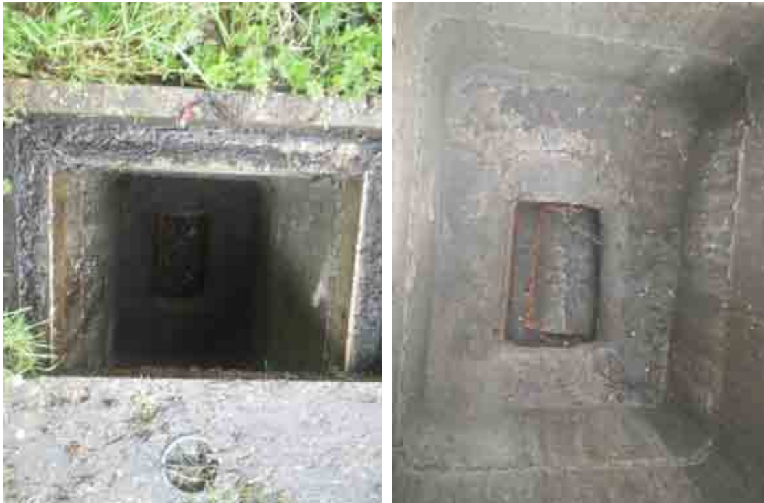
Figure 5-4: Manholes to the south of Craignee Drive
