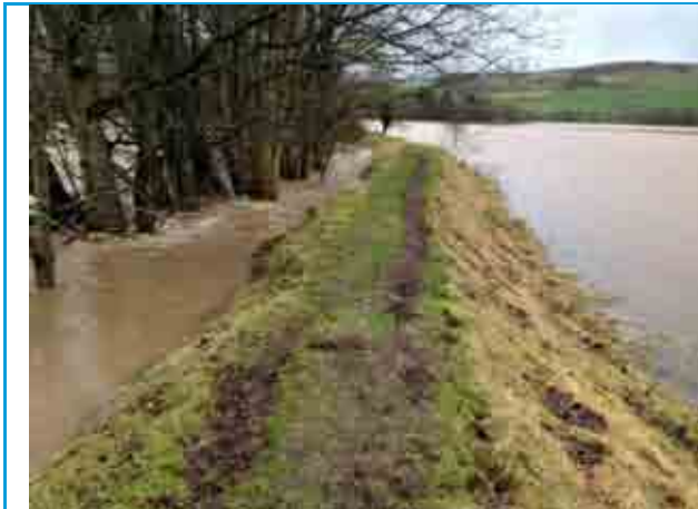
Ponded flood water in floodplain downstream of footbridge
