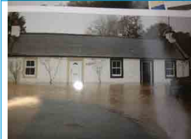
Flooding on Dunreggan Brae adjacent to High Street Bridge
