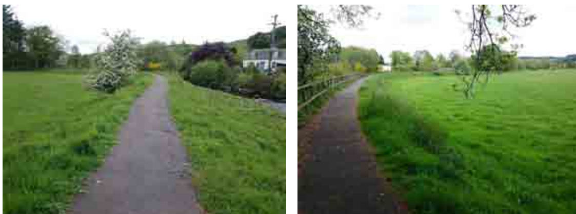
Figure 7-6: Embankment in downstream reach (Assets 7 & 8)
