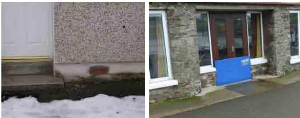
Figure 7-1: Examples of PLP (automatic airbrick and door guard)
