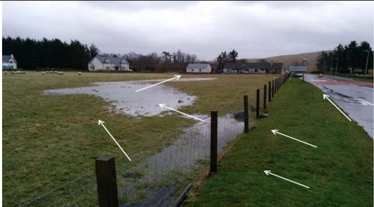
Photo 9: Flow path of water overtopping A713 (Jan 15)
