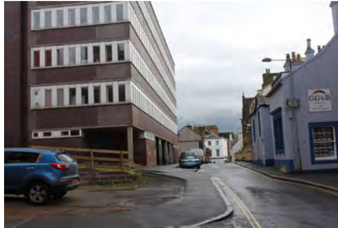
Irish Street - before and after
