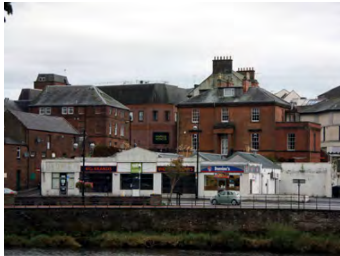
Whitesands gap site - before and after
