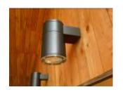
A fully cut-off light fitting making a downward cone of light with no stray light. This fitting illuminates a doorway only. This light fitting does not have additional shielding and therefore viewed light may be seen from a distance if in a rural setting but may not be problematic if the light source is less than 1,000 lumens. Front facing shields are available if needed.
