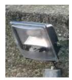
Many rural properties such as steadings, milking sheds, yards and even houses have flood lights such as this and they often give off a bright orange light. The reflector unit held within the light fitting is bi-symmetric and should be installed facing directly downward. However, the unit also has a curved glass panel on the front to aid with light spread which means even pointing directly downward it will still have an upward stray light content. This is not supportive of the Dark Sky Park.
